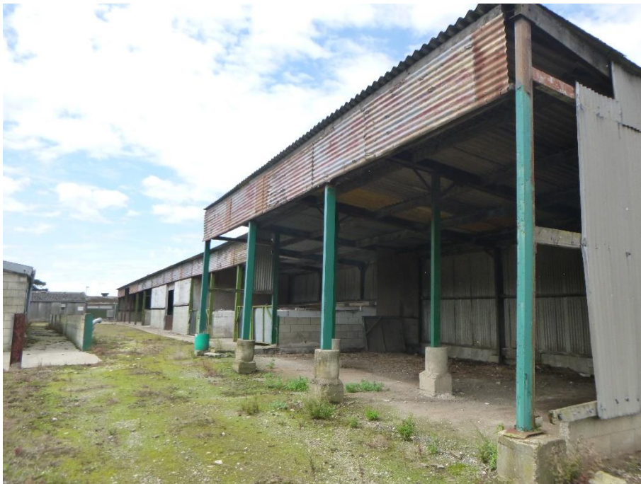
Plate 4: View of central part of piggery. Facing west.
