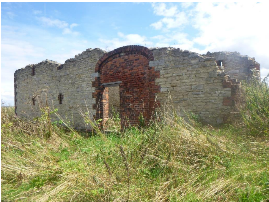
Plate 8: Appleby Carr Farmstead (MLS25147). This Post-medieval farm was established on the site of Thornholme Augustinian priory after the dissolution. It now forms the most visually obvious remains within the area of the Priory Scheduled Ancient Monument. Facing south-east.
