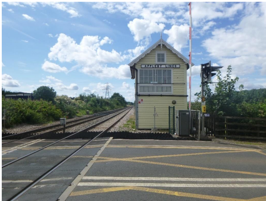
Plate 6: Appleby Signal Box (NHLE 1161513; MLS9195). View of immediate setting showing the relationship between the asset, the railway, the B1207 road and the level crossing. Facing west.
