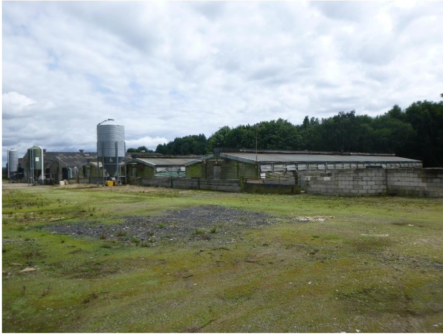
Plate 3: View of south-eastern part of piggery, including (nearest camera) 3 no. buildings to be demolished. Facing south-east.
