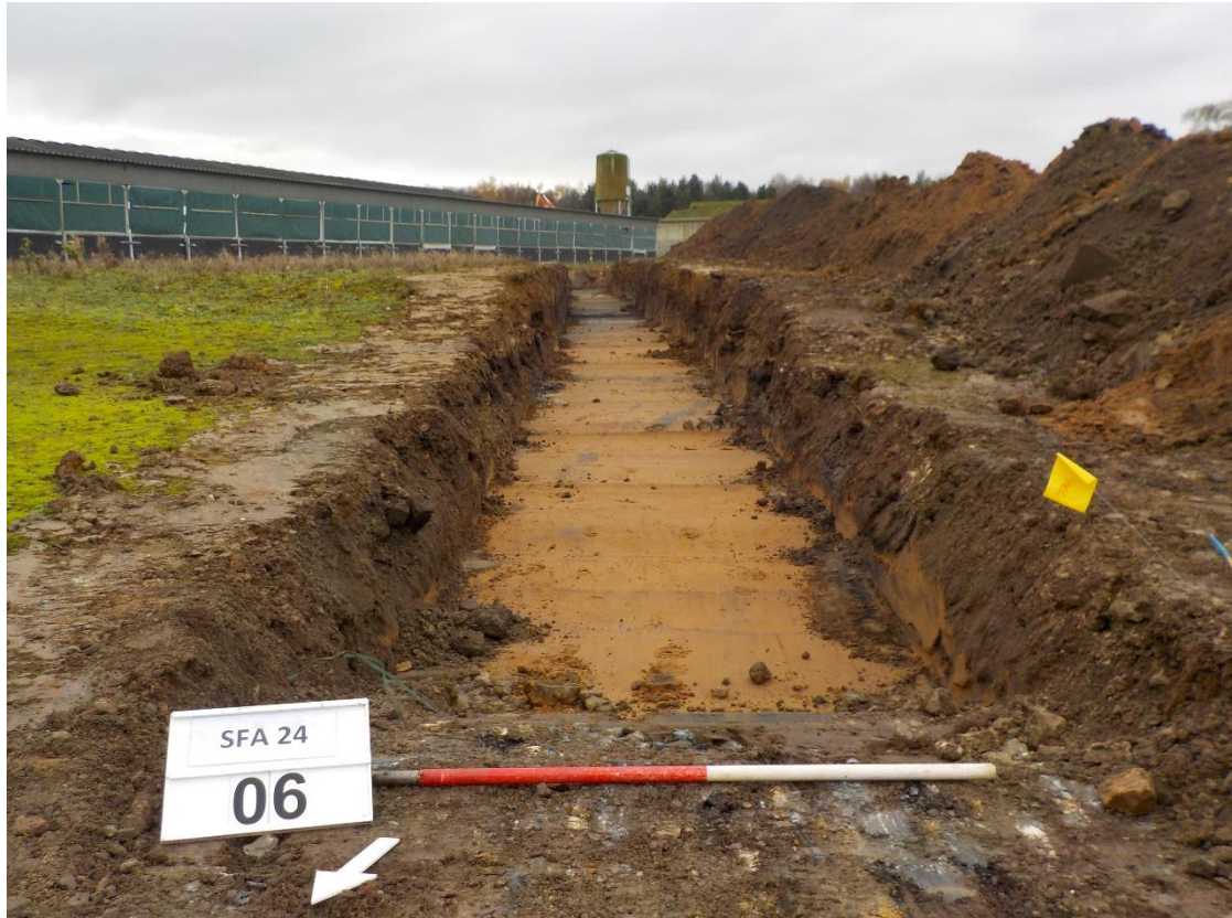
Plate 9: Trench 06 camera facing south-south-east
