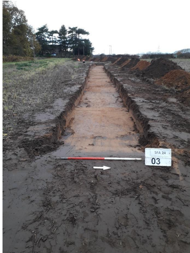
Plate 3: Trench 03 camera facing east
