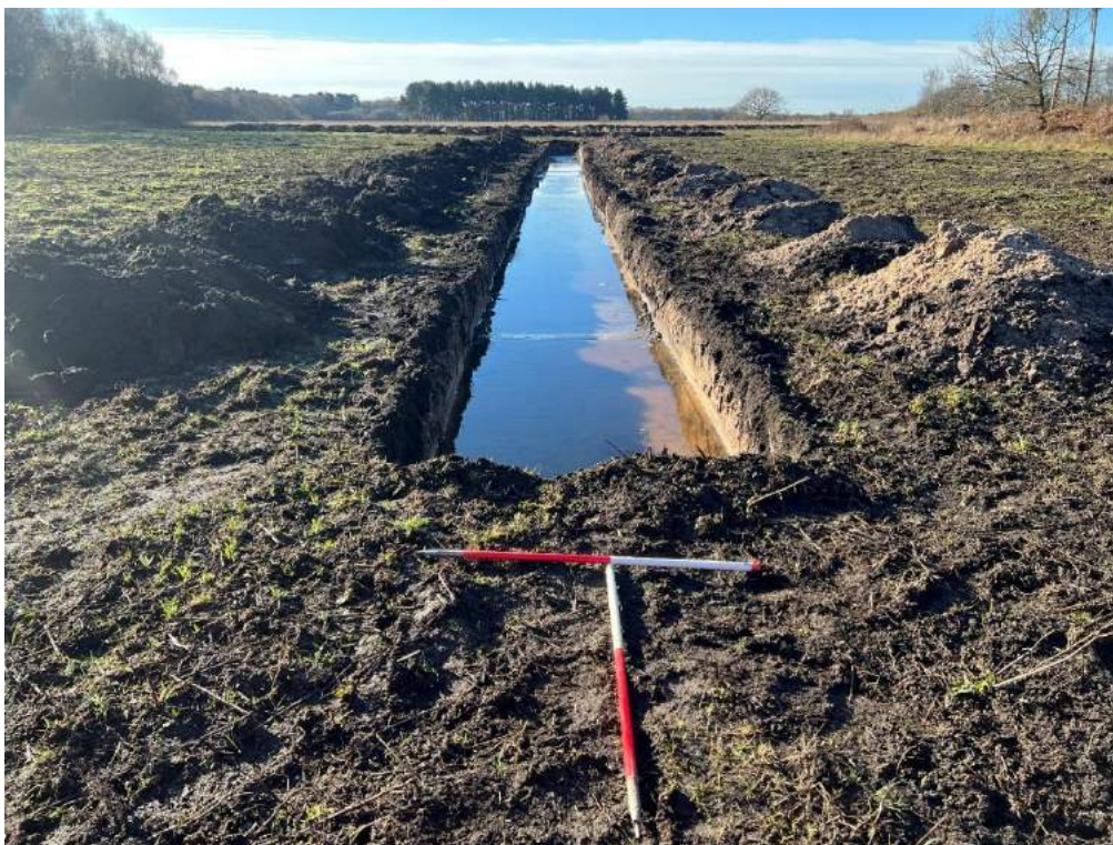
Plate 5: Trench 03, overall shot
