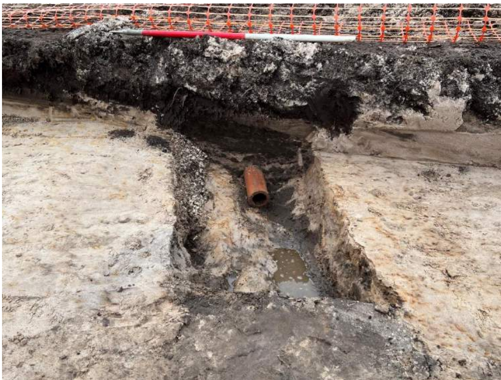
Plate 15: Potential archaeological feature in trench 04, proven to be a land drain.
