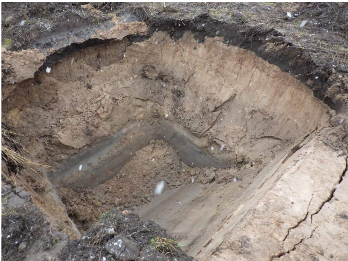
Plate 29: Test Pit 4 (TP04) carried out at the western end of Trench 4. Collapse at 2.10m BGL.
