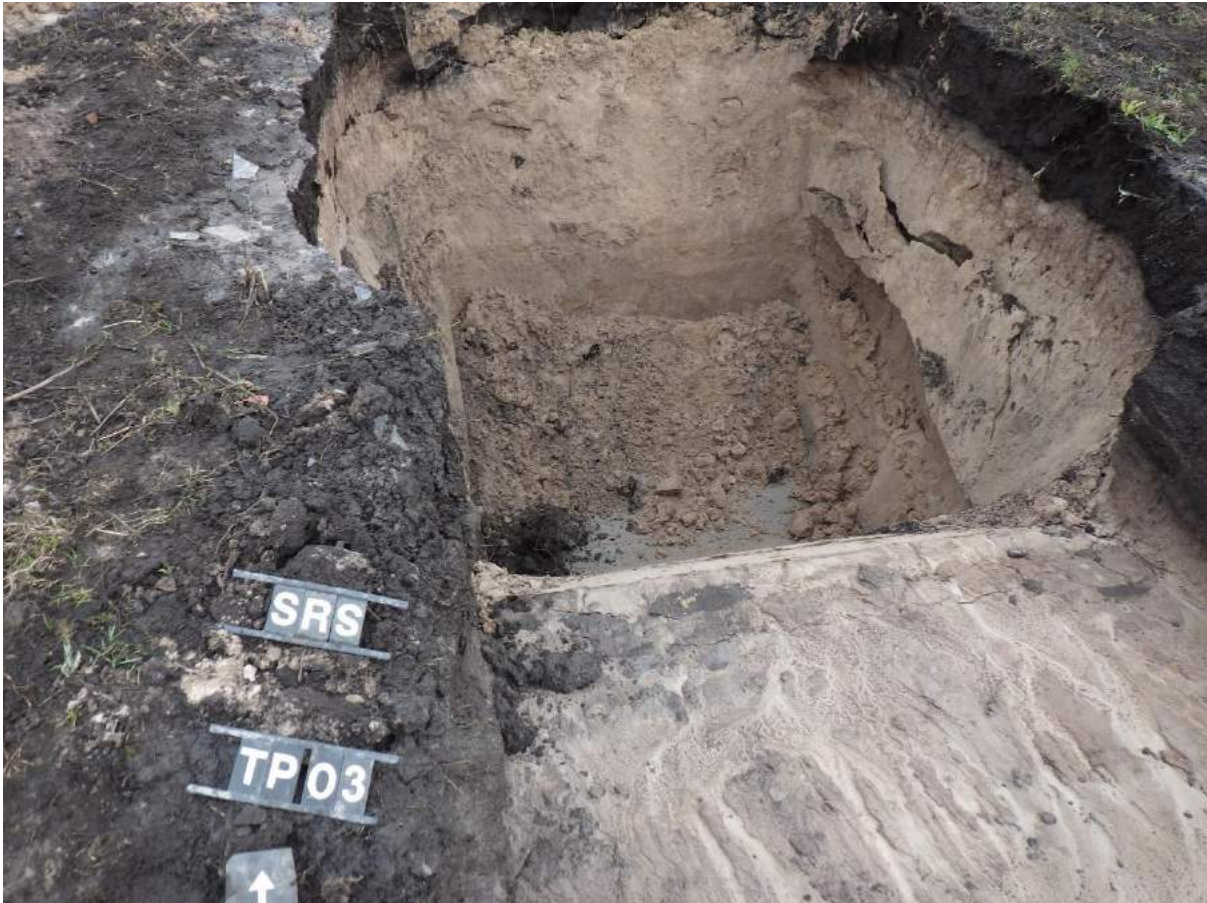
Plate 25: Test Pit 3 (TP03) carried out at the northern end of Trench 3
