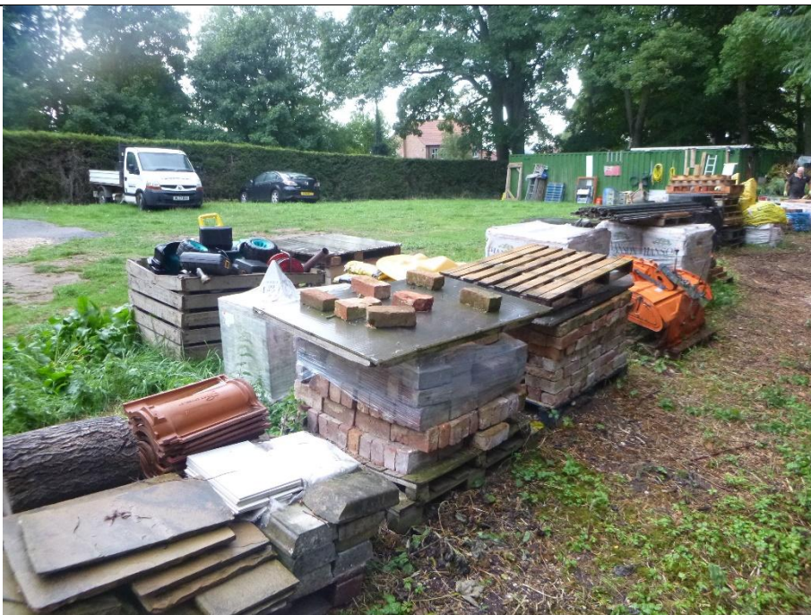
Site Photo: 13 Date: 06 Sep 2022 Photo direction: South Description: Construction materials stored inside the northwest site boundary
