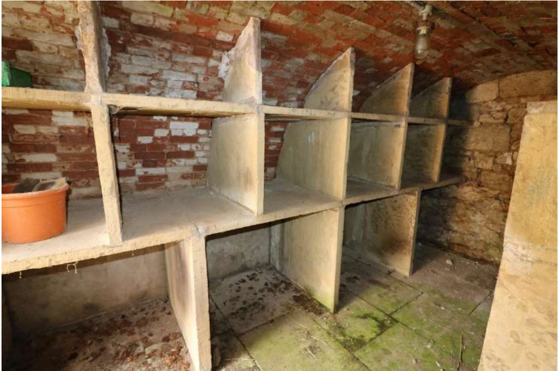
Figure 52 The interior of Chamber 2
