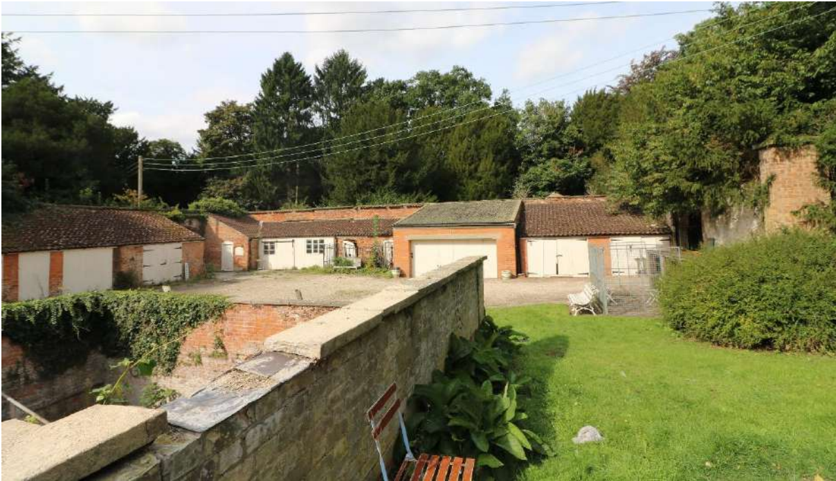
Figure 58: General view of the courtyard outbuildings looking north west
