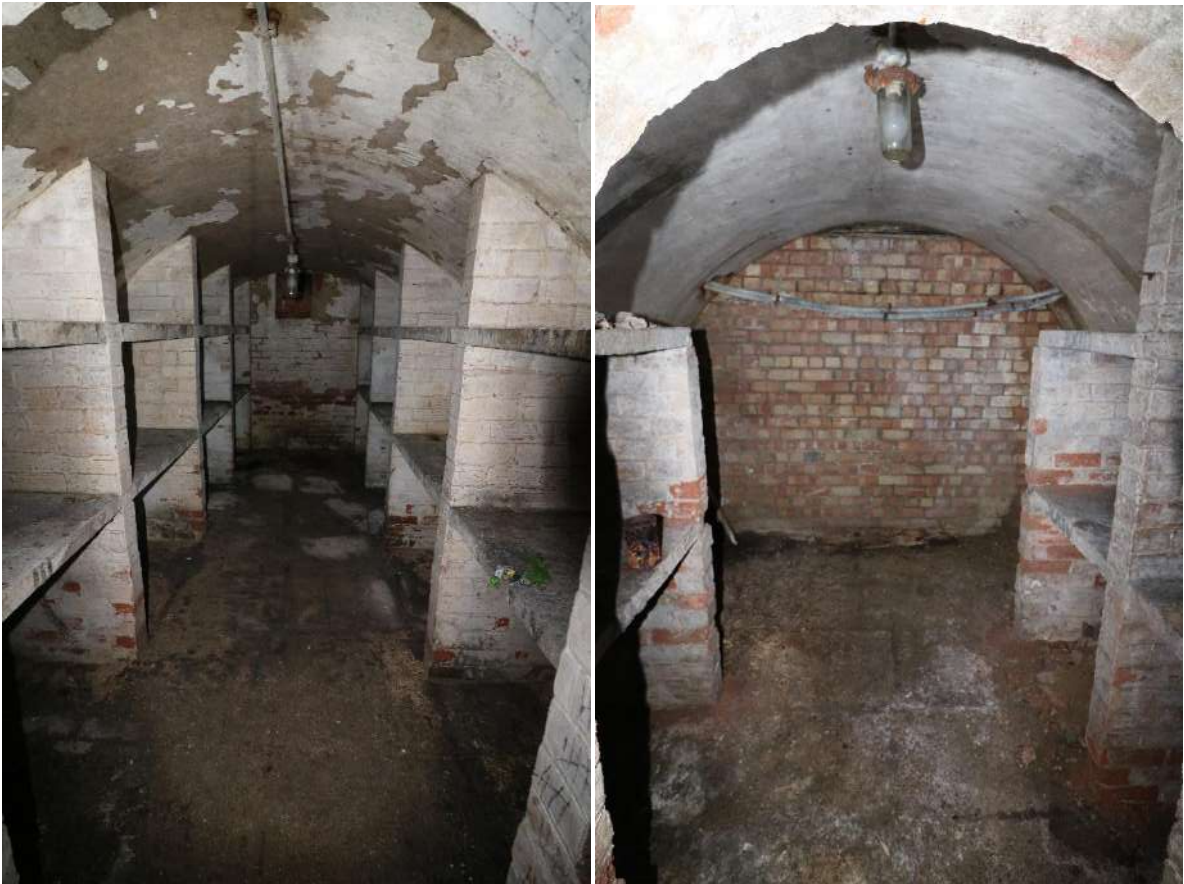
Figure 55 Chamber 3 looking north (left) and Chamber 4 looking south (right).
