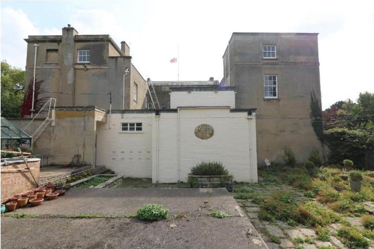
Figure 43 The north elevation of Elsham Hall in the present day.
