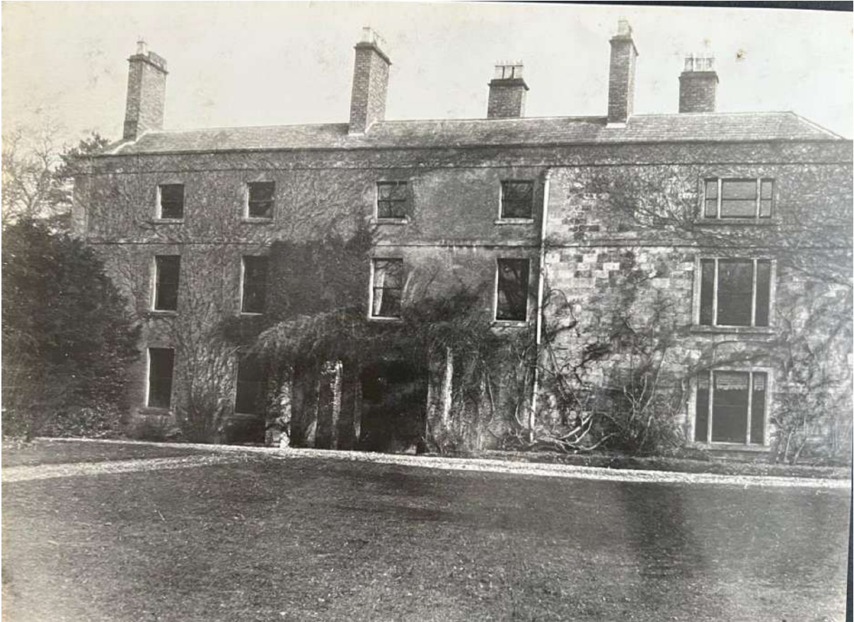
Figure 24: Likely early 20th century photograph of the western elevation of Elsham Hall showing the two different phases of the extension, seen on Site visit on 22/09/22
