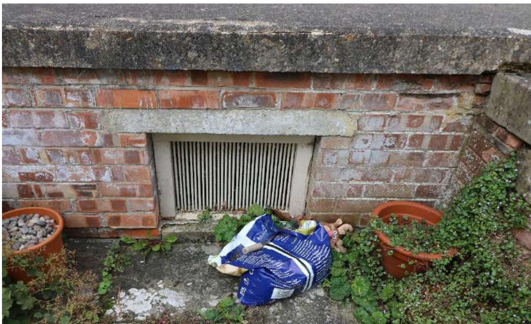
Figure 32: The air vent at the rear of cellar Chamber 2. Note the projection above ground level and the concrete capping over.
