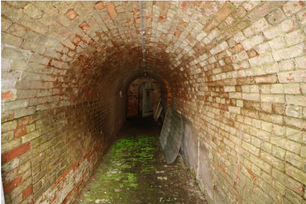
Figure 53 The cellar corridor
