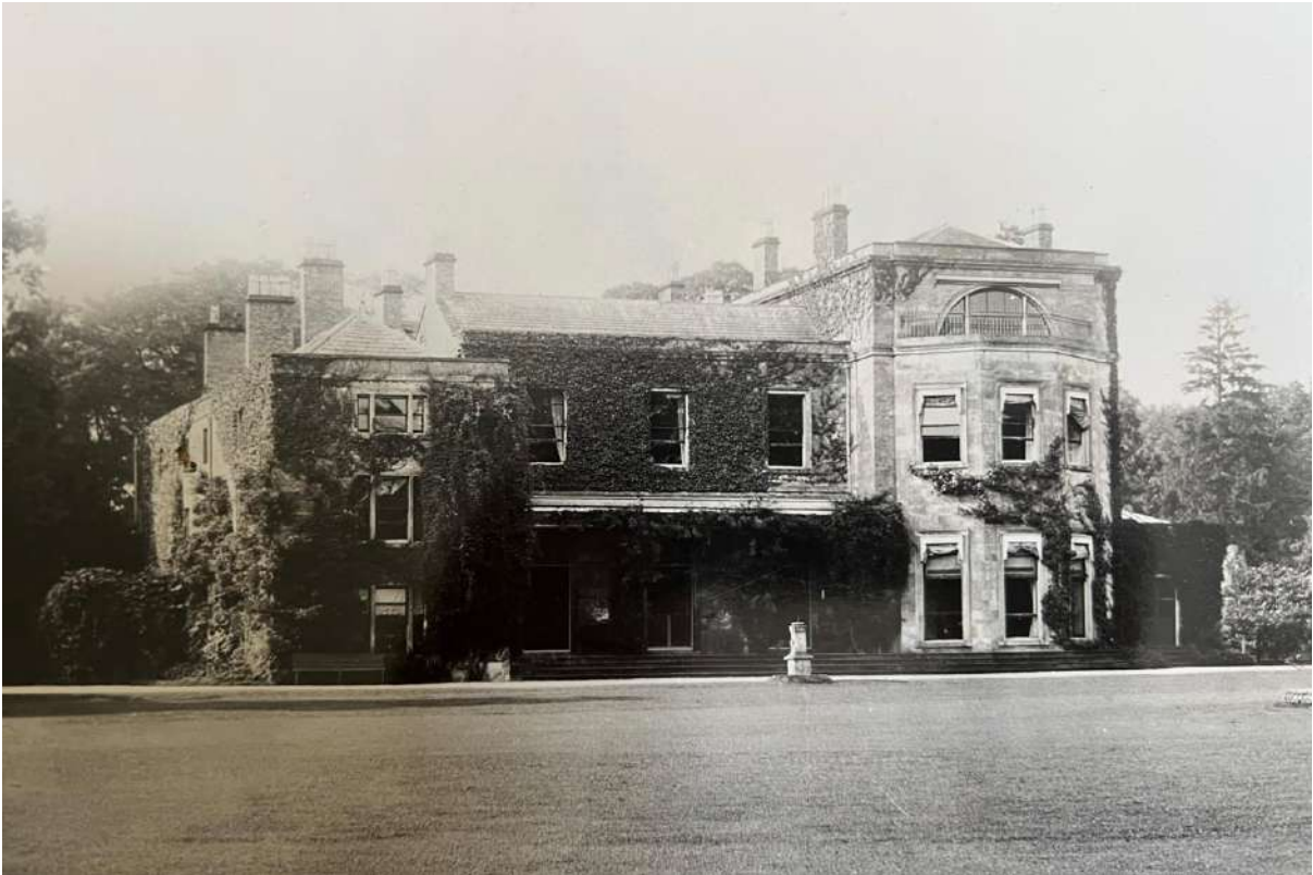
Figure 23: Likely early 20th century photograph of the south elevation of Elsham hall showing the 19th century changes to the hall, seen on Site visit on 22/09/22
