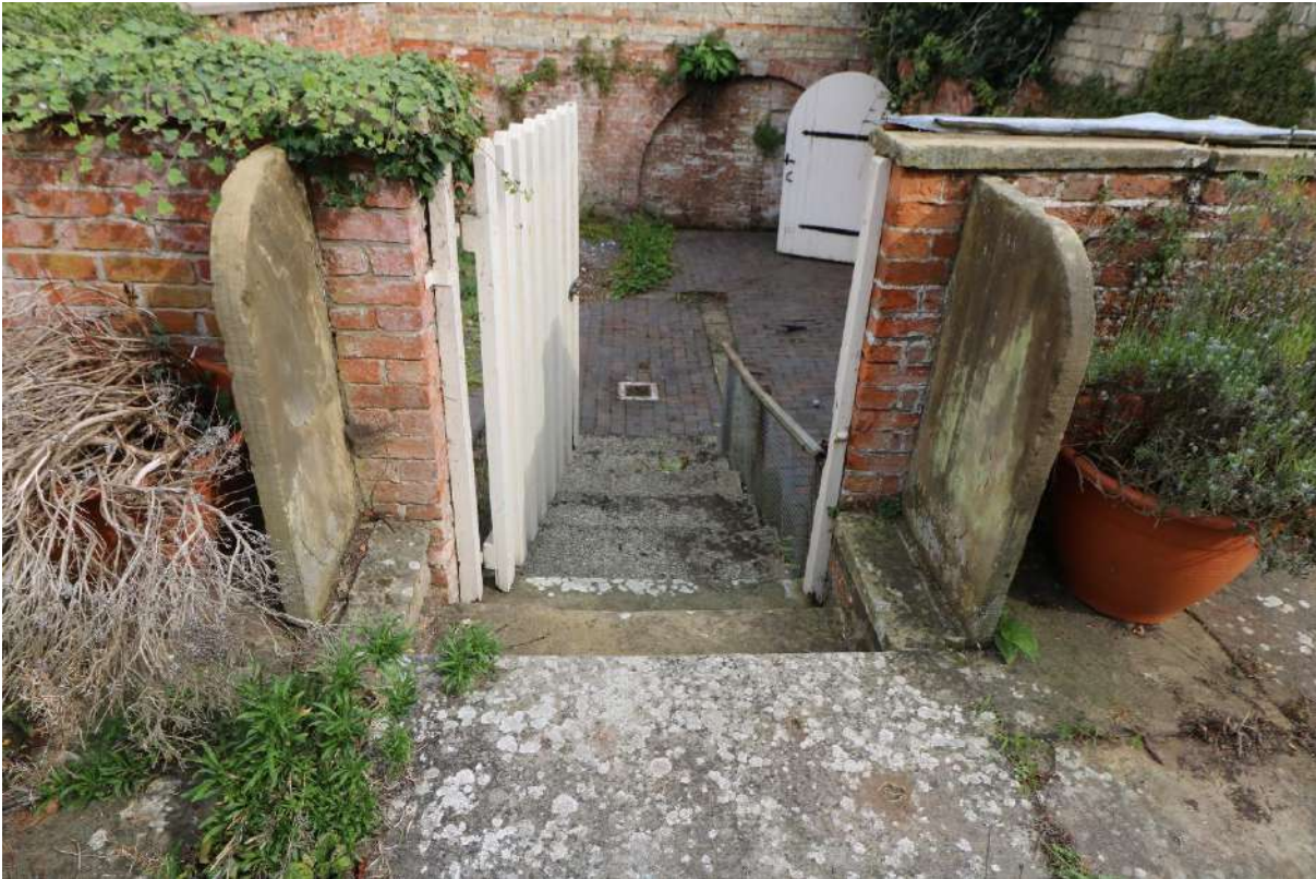
Figure 35: The entrance gate at the west end of the wash yard.
