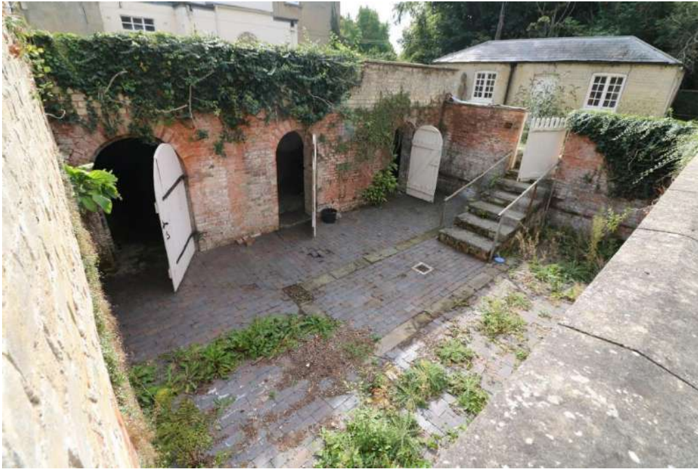
Figure 45 View over the wash yard looking south west.
