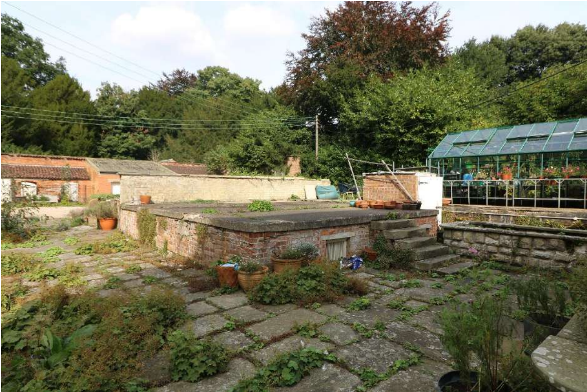
Figure 37: View north east over the concrete capped cellars.
