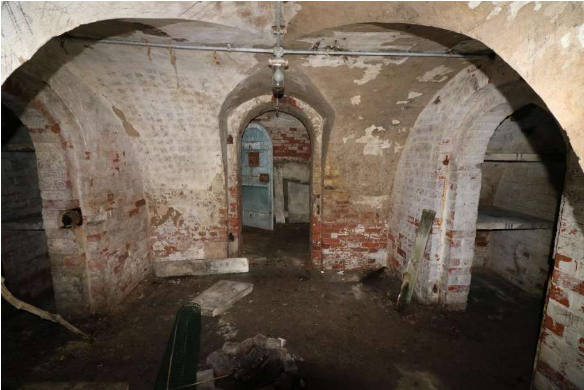
Figure 54 The cellar lobby looking west towards the corridor.
