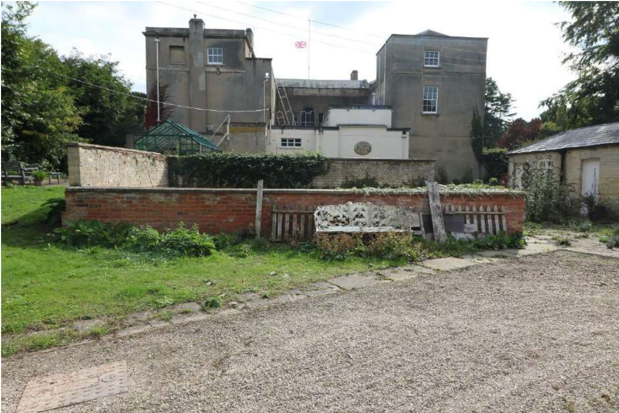
Figure 34: View south towards the north elevation of the Hall. The low wall in the foreground forms the parapet to the sunken wash yard.
