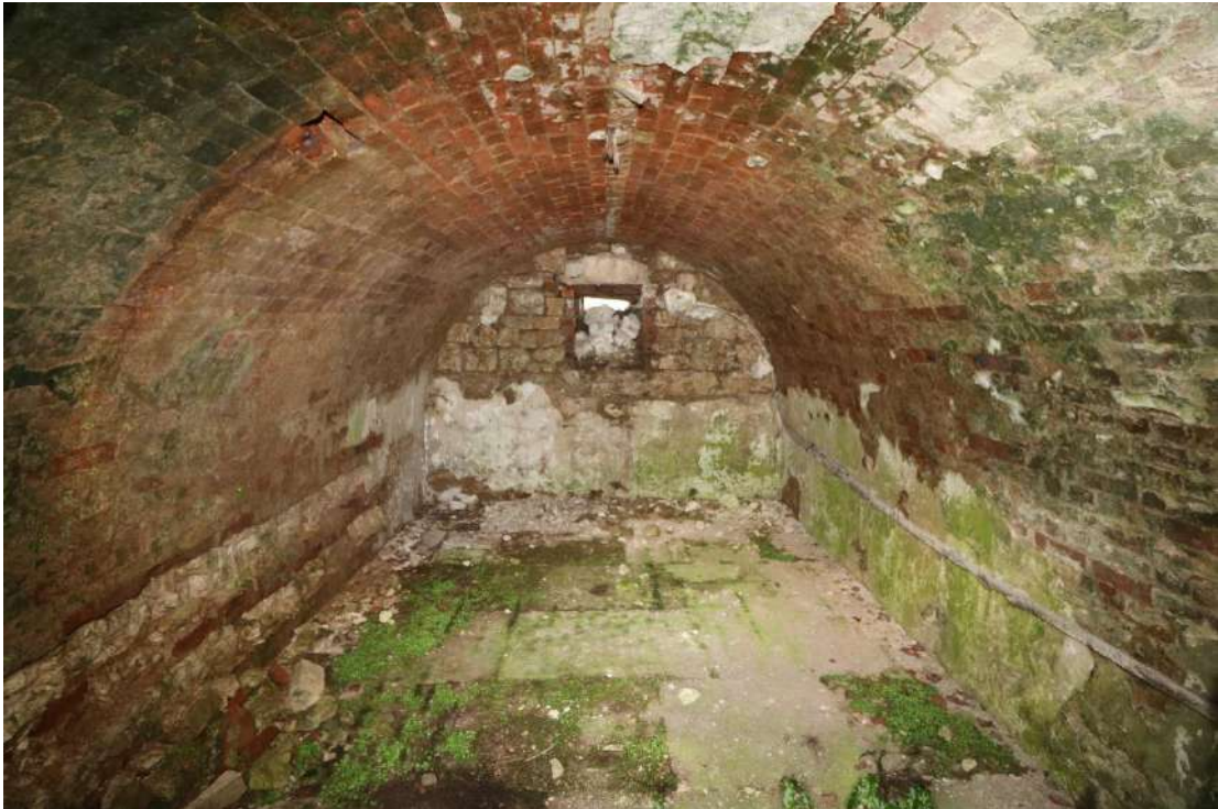
Figure 51 The interior of Chamber 1
