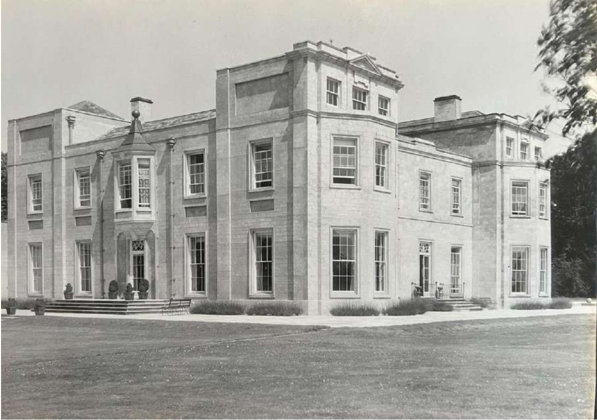
Figure 27: Western and southern elevations of Elsham Hall after the 1930s alterations, seen on Site visit on 22/09/22
