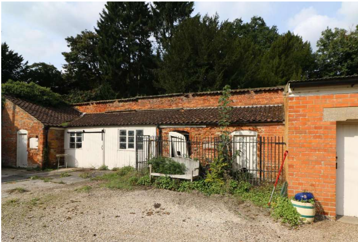
Figure 60: Outbuildings in the north west corner of the courtyard
