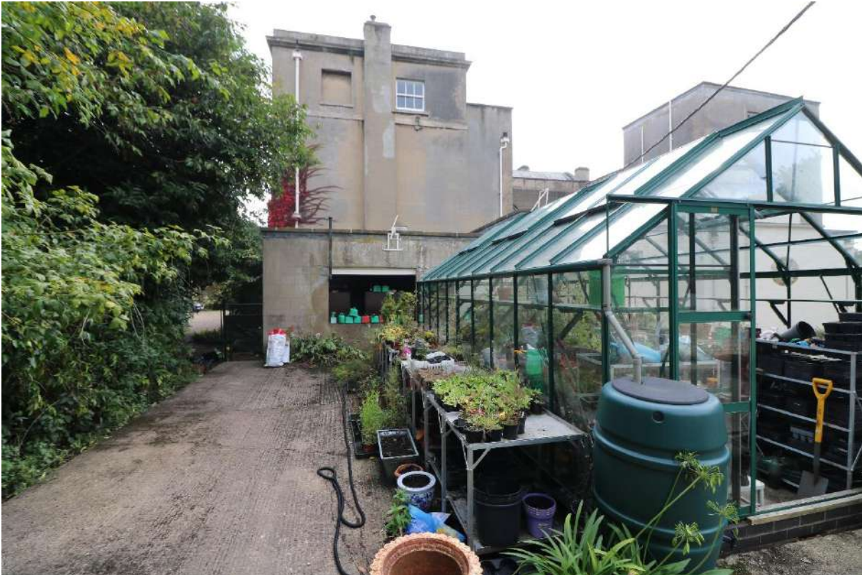
Figure 38: The boiler room and oil store at the north end of the east wing.
