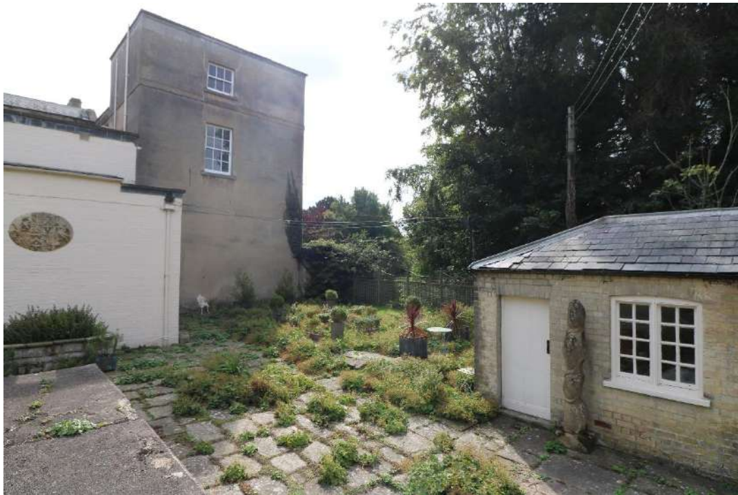
Figure 31: The position of the demolished north west service wing. The single storey building to the right is a 19 th century game store.
