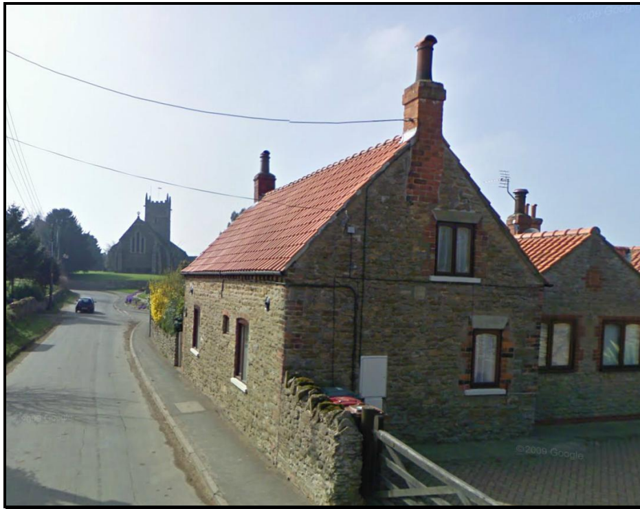
Early Single Storey Stone Cottage
