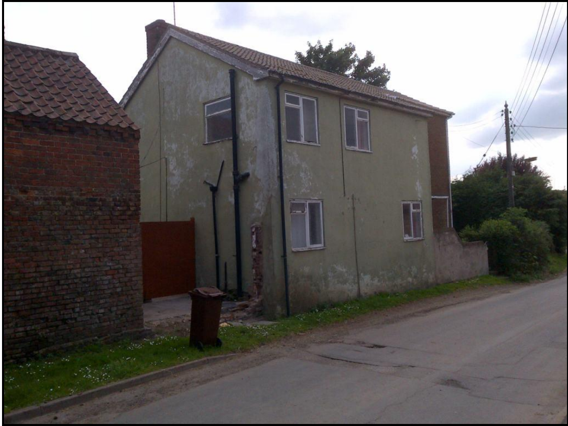
North Elevation onto Whitton Road
