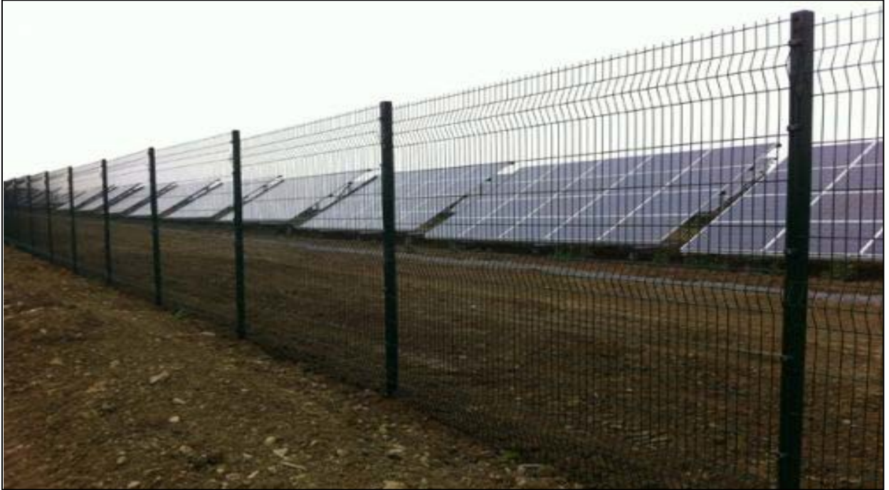
Plate 3 Example of Security Fencing
