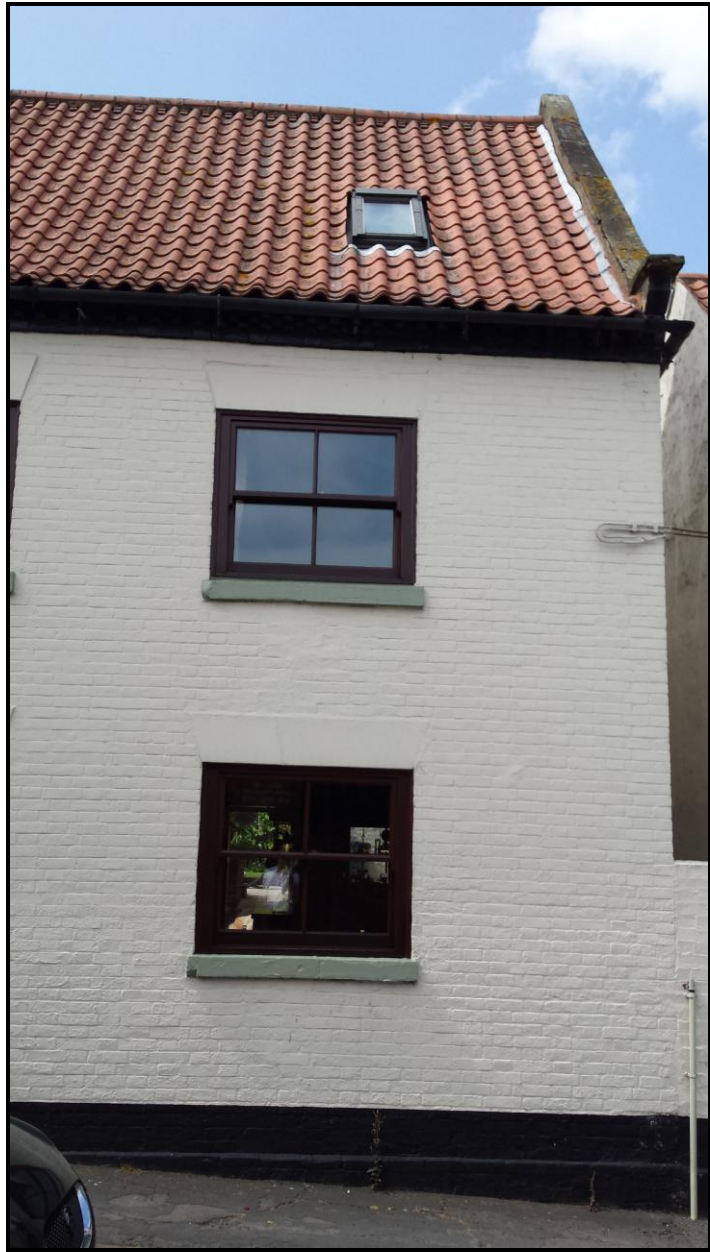
Northern End of East Elevation
