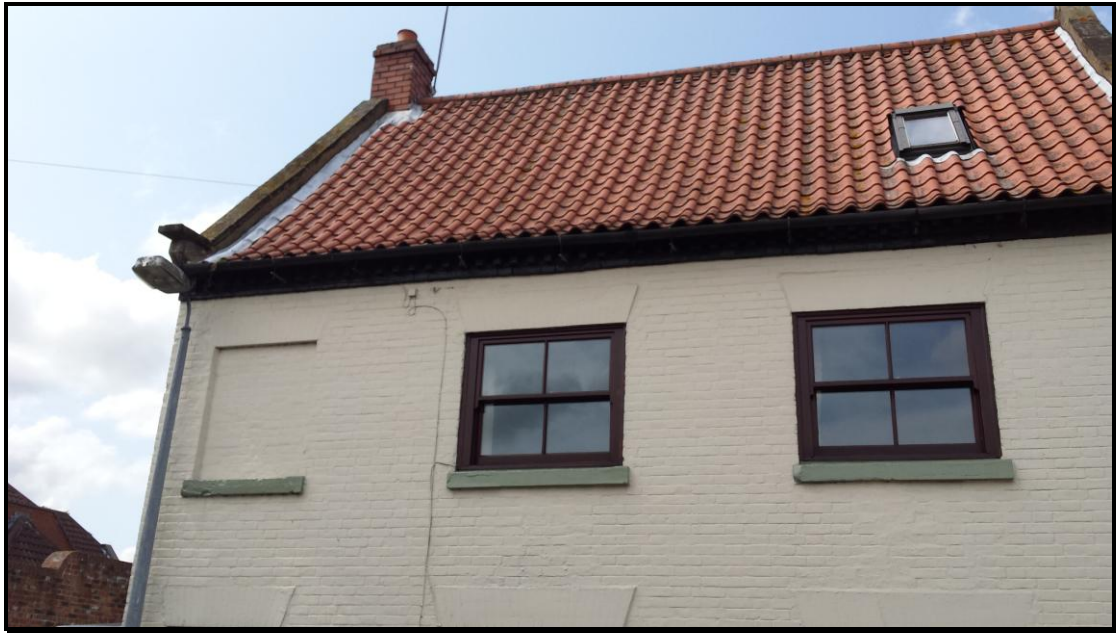
East Elevation, High Level, of Property
