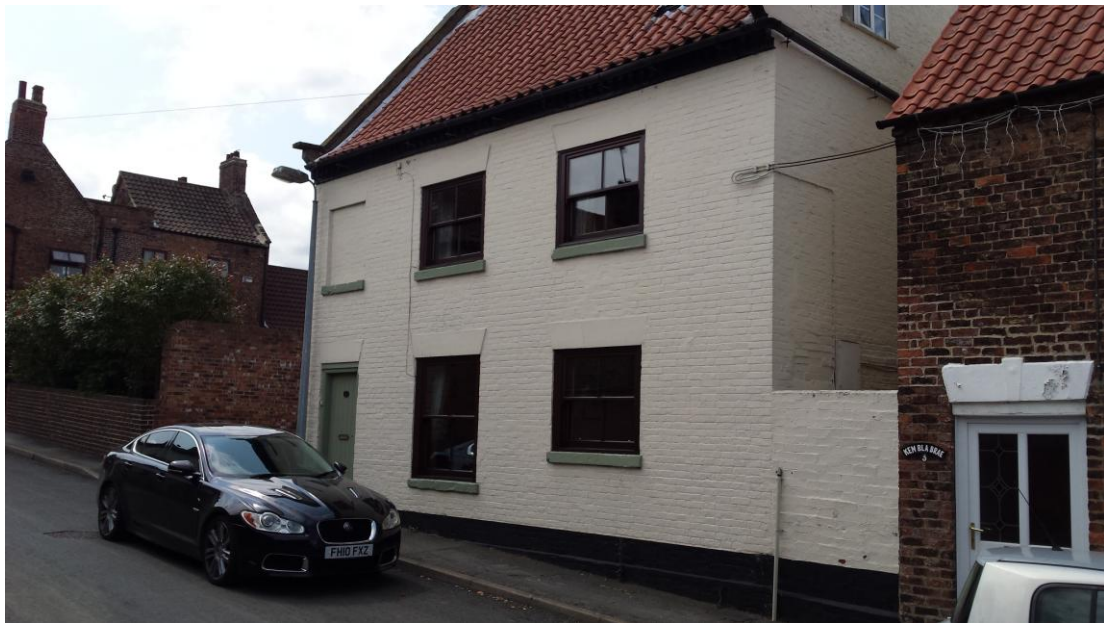
East Elevation, Low Level, of Property
