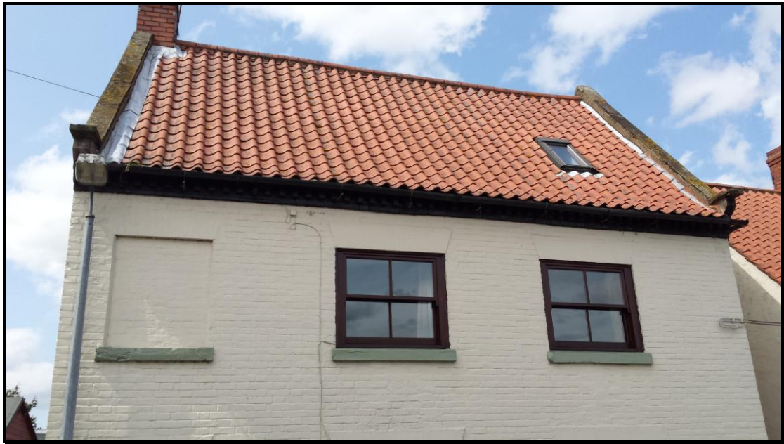
East Elevation, High Level, of Property
