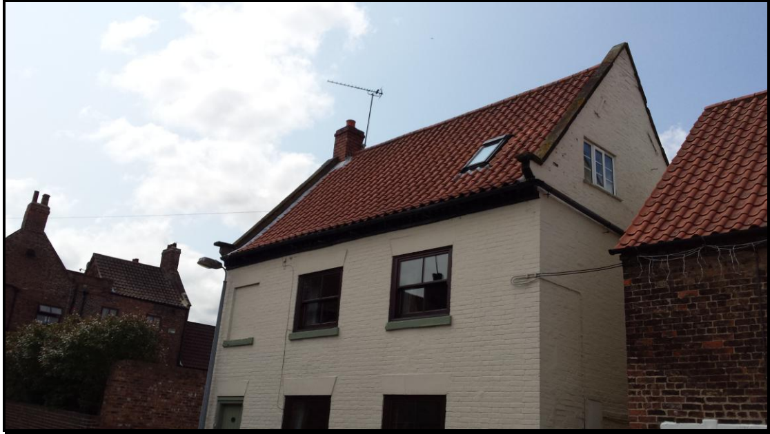
East Elevation, High Level, of Property
