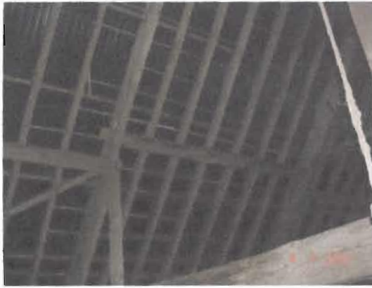
Fig. 2 Interior of barn upper floor.
