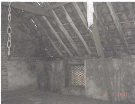
Fig. 3 Interior of granary upper floor.
