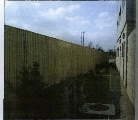
2.5m high barrier at waterworks
