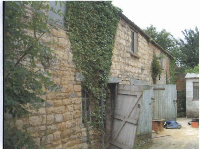
Plate 2 Front elevation of the Barn (as viewed from the north-east).
