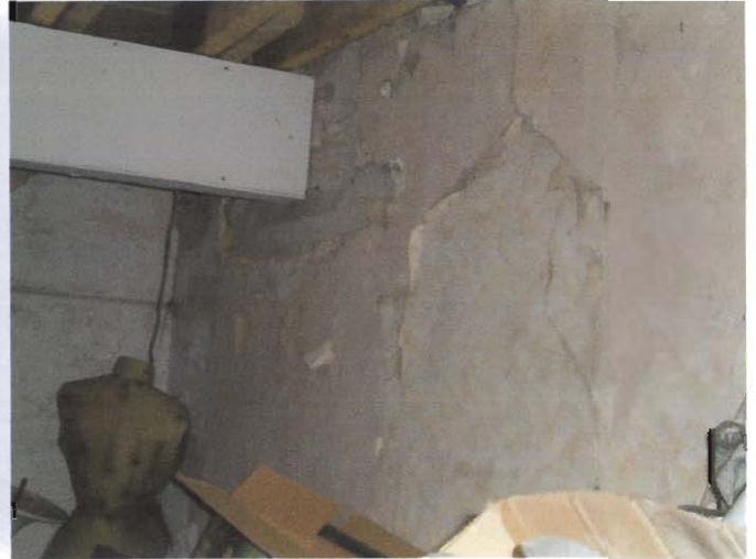
Plate 14 Room 2 (west wall)
