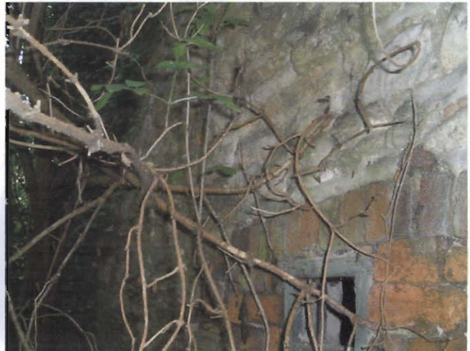
Plate 4 East Elevation of the barn (at low level within passageway).
