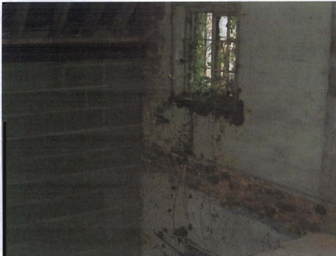
Plate 9 First floor (view on western gable wall).
