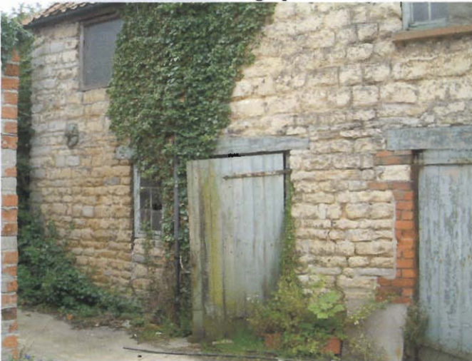
Plate 1 Front (north) elevation of the Barn (left hand side).
