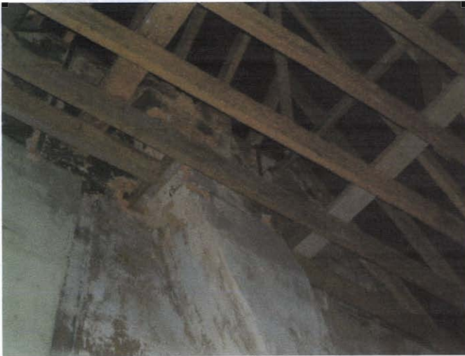
Plate 13 Exposed roof timbers as viewed from ground floor level.
