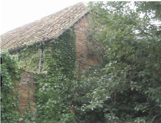
Plate 5 West Elevation of the barn (again partially obscured by vegetation).
