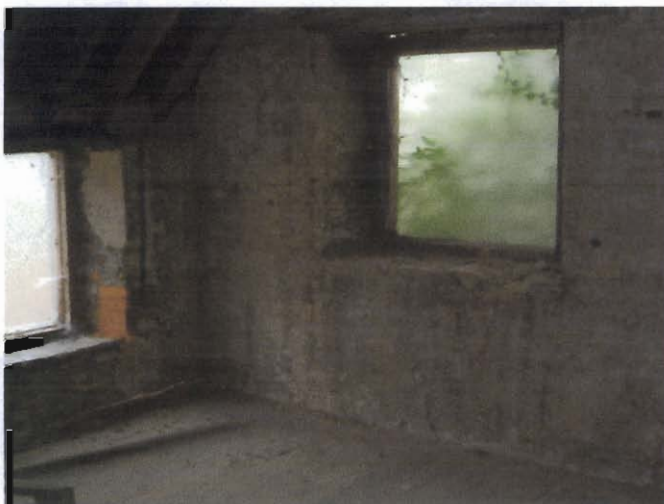
Plate 11 First floor (north-east corner of main room).
