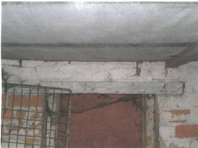
Plate 15 Roof panelling over doorway to Building 3.
