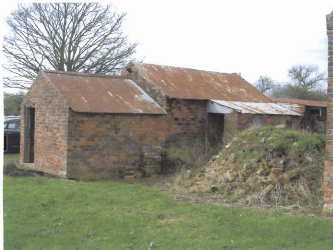
Plate 9 Northern elevation of Building 2.
