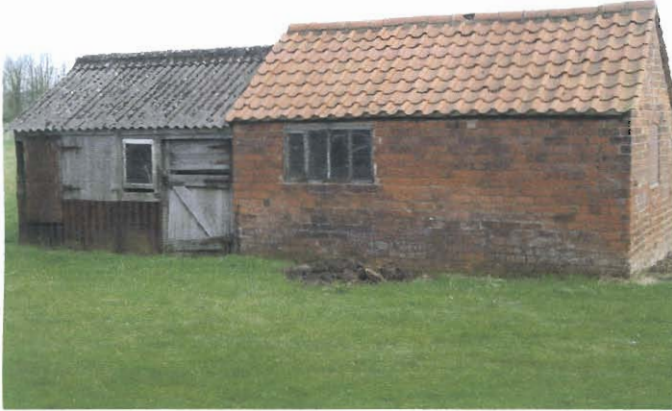
Plate 13 Western elevation of Building 3.
