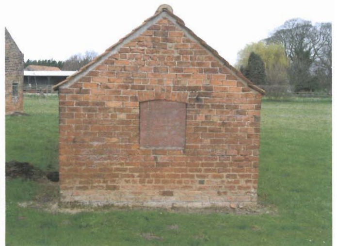
Plate 14 Southern elevation of Building 3.
