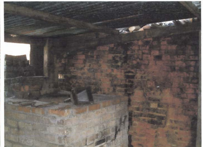
Plate 10 Western elevation of Building 2 (from within storage area).
