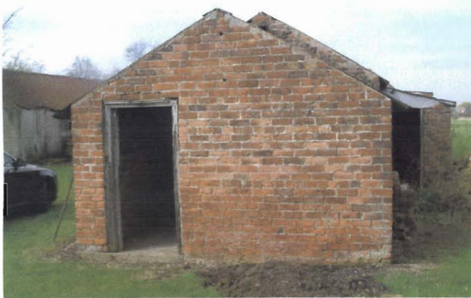
Plate 7 Eastern elevation of Building 2.
