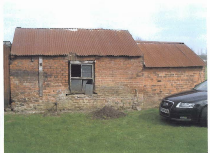
Plate 8 Southern elevation of Building 2.
