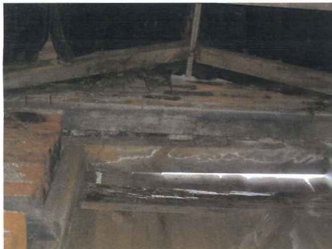
Plate 5 Roof structure over the western gable wall of the barn.
