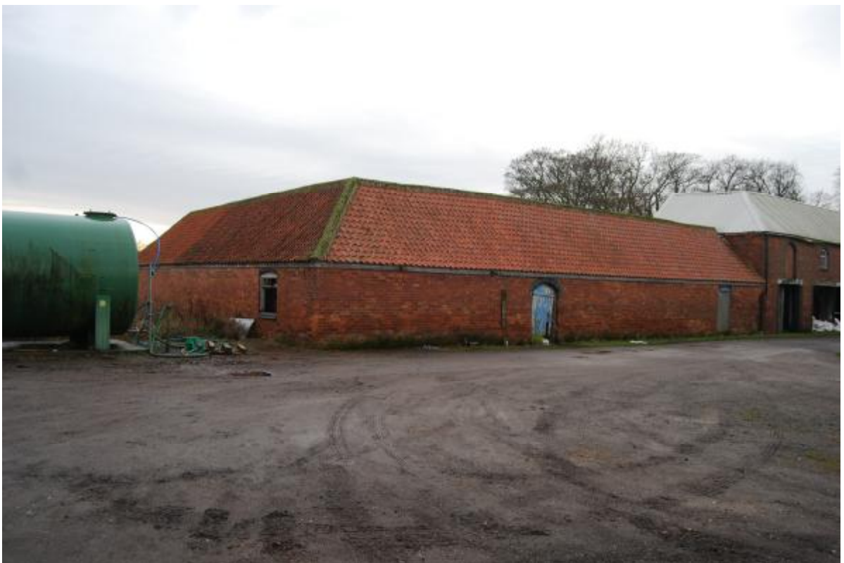
View to south west of the site, adjacent buildings
