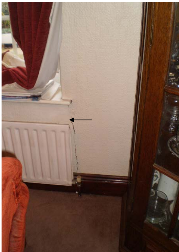
Rear ground floor sitting room – right flank
