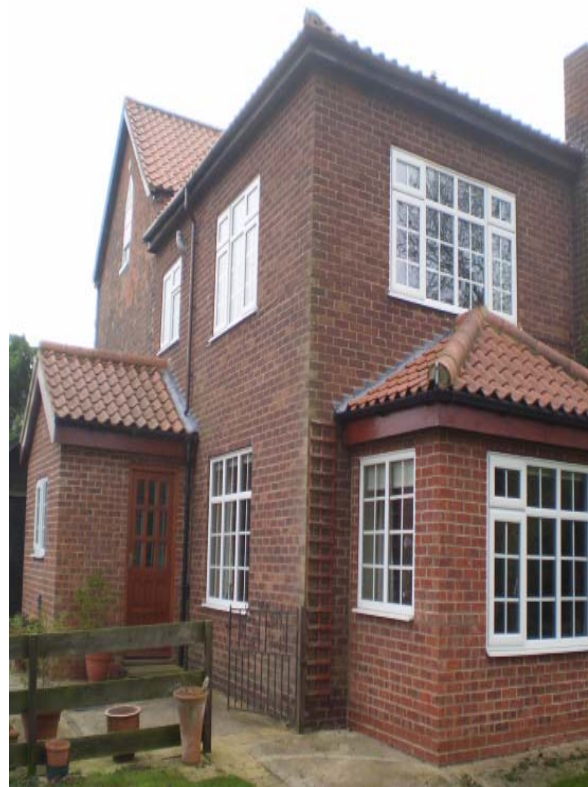
View of extension right hand flank
