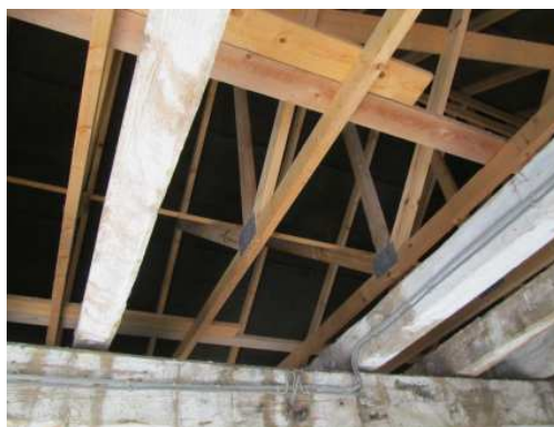
Fig.6. Interior of roof in Building C.
