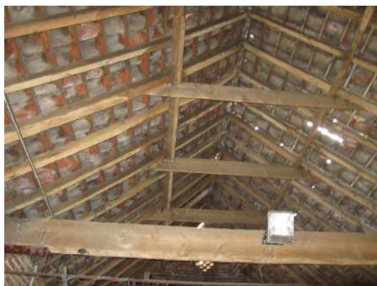
Fig.3 Roof of Barn A.
