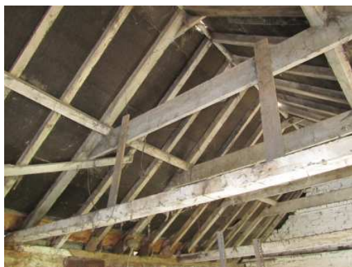
Fig. 5 Interior of roof in Building B.
