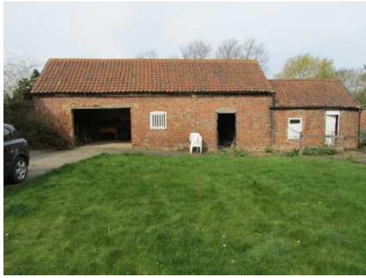
Fig.1 Western range. Building C.
