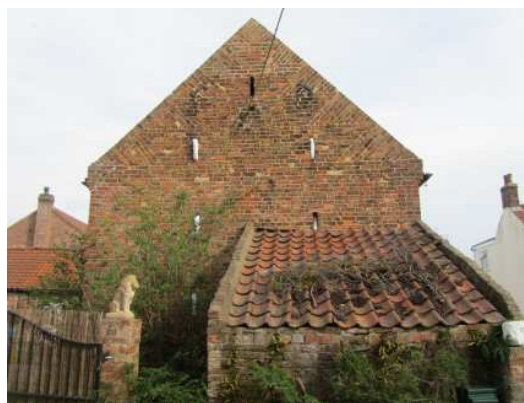
Fig.4 South gable and lean-to Building A.
