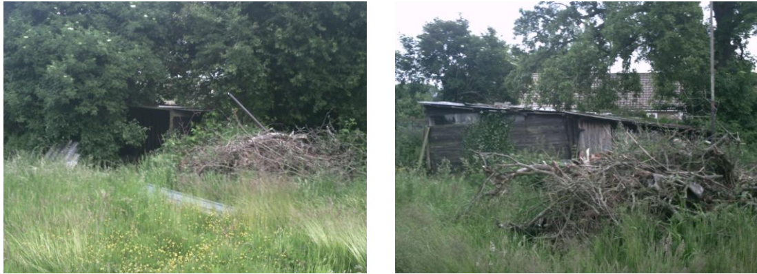
Photograph 3: Log store (left) and Poultry building 1 (right)
