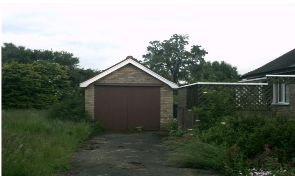
Photograph 2: Garage – northern aspect.
