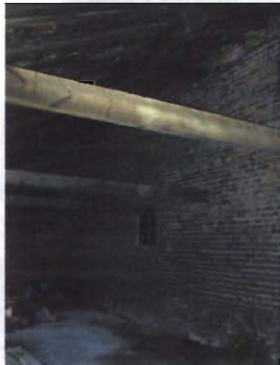
E. North elevation under catslide roof
