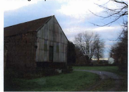
D. North elevation – corrugated tin sheeting to open-ended barn
