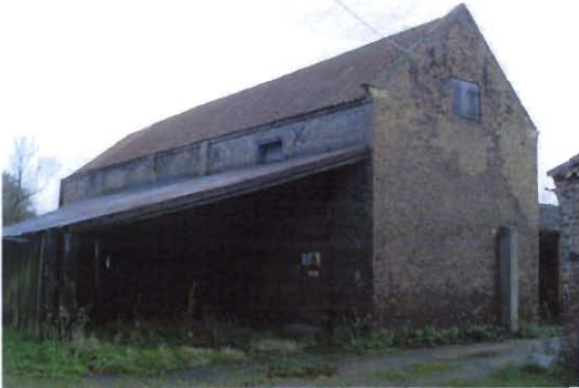
G. North elevation – corrugated tin sheeting to open-ended barn
