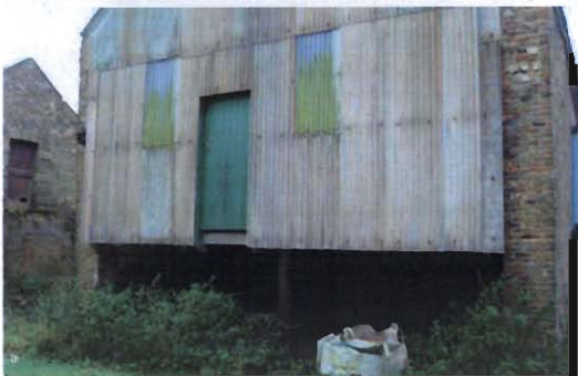
G. North elevation – corrugated tin sheeting to open-ended barn
