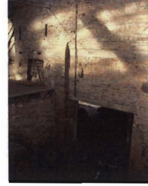
D. Blocked up arched opening from above
