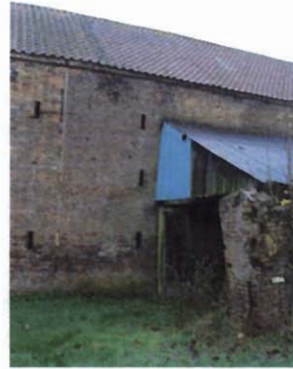
C. Lean-to shed
