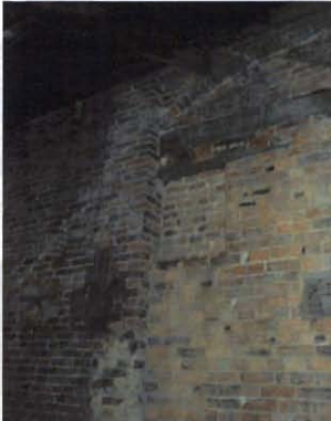
F. Blocked up arched opening
