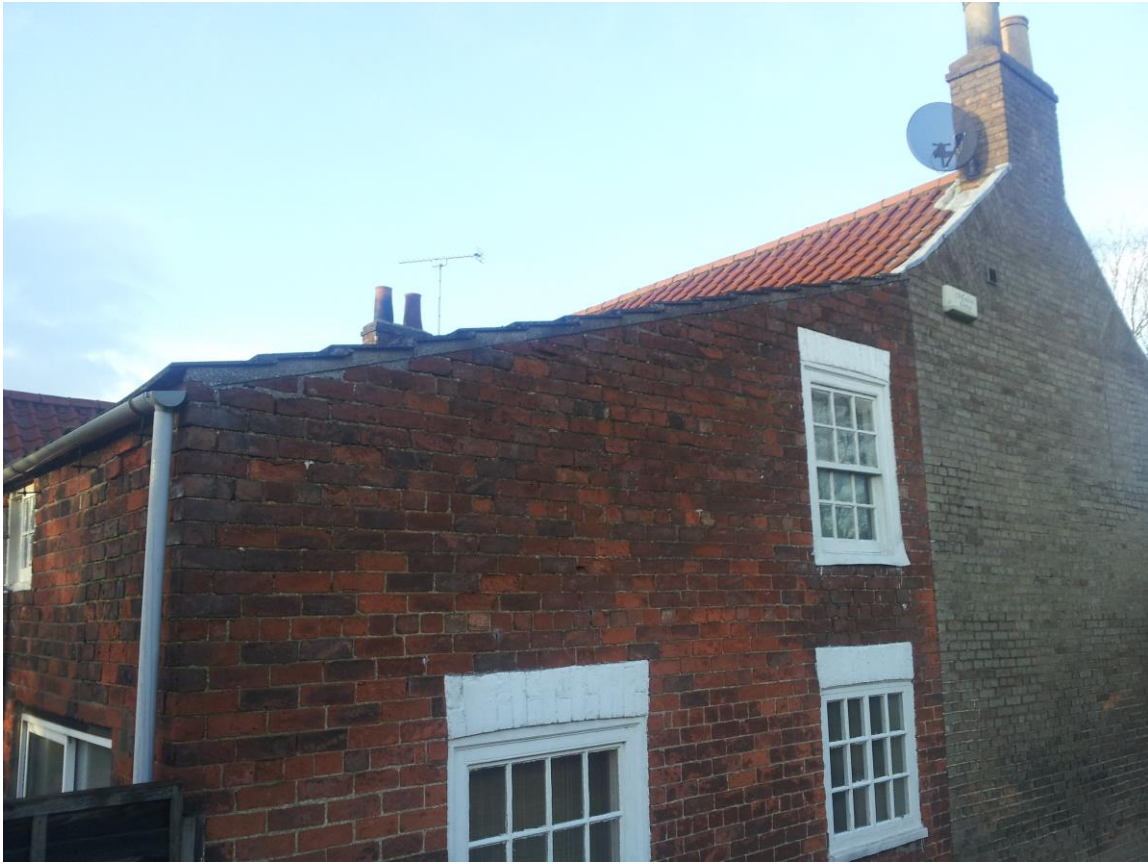
East Elevation showing the extension
