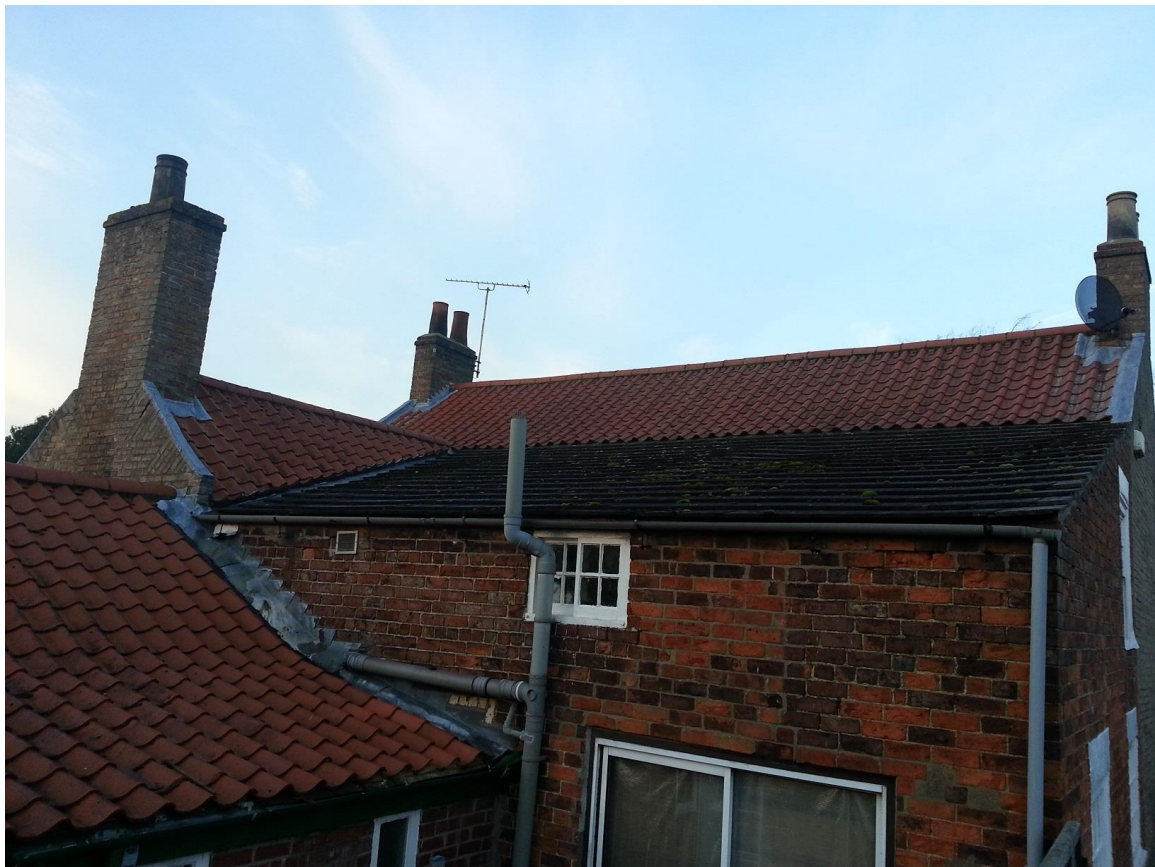
Rear Elevation showing concrete roof tiles and Aluminium Patio Door.
