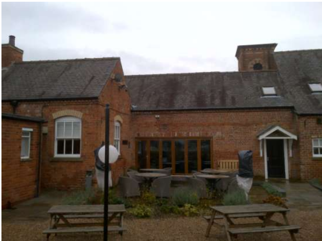
North West Elevation - Looking North East
