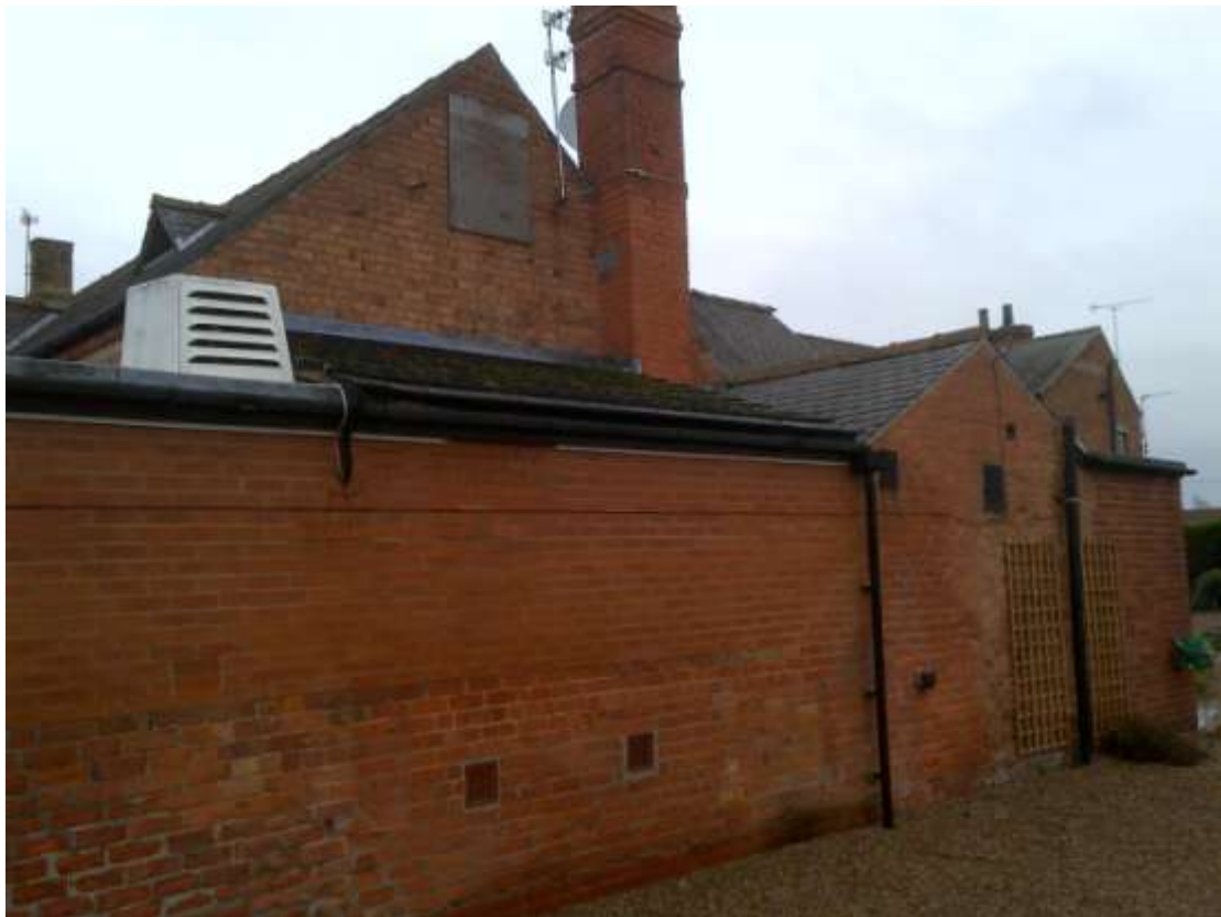
North West Elevation - Looking South East
