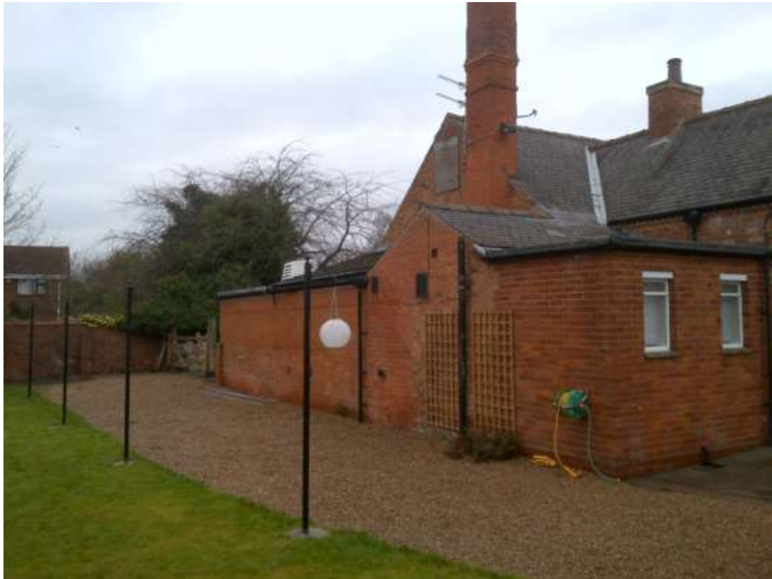
North West Elevation - Looking North
