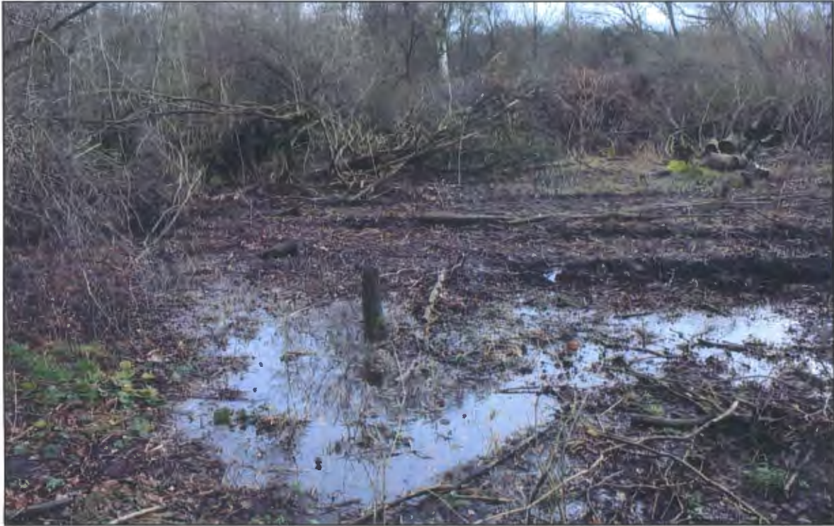
Plate 9. Areas of standing water.
