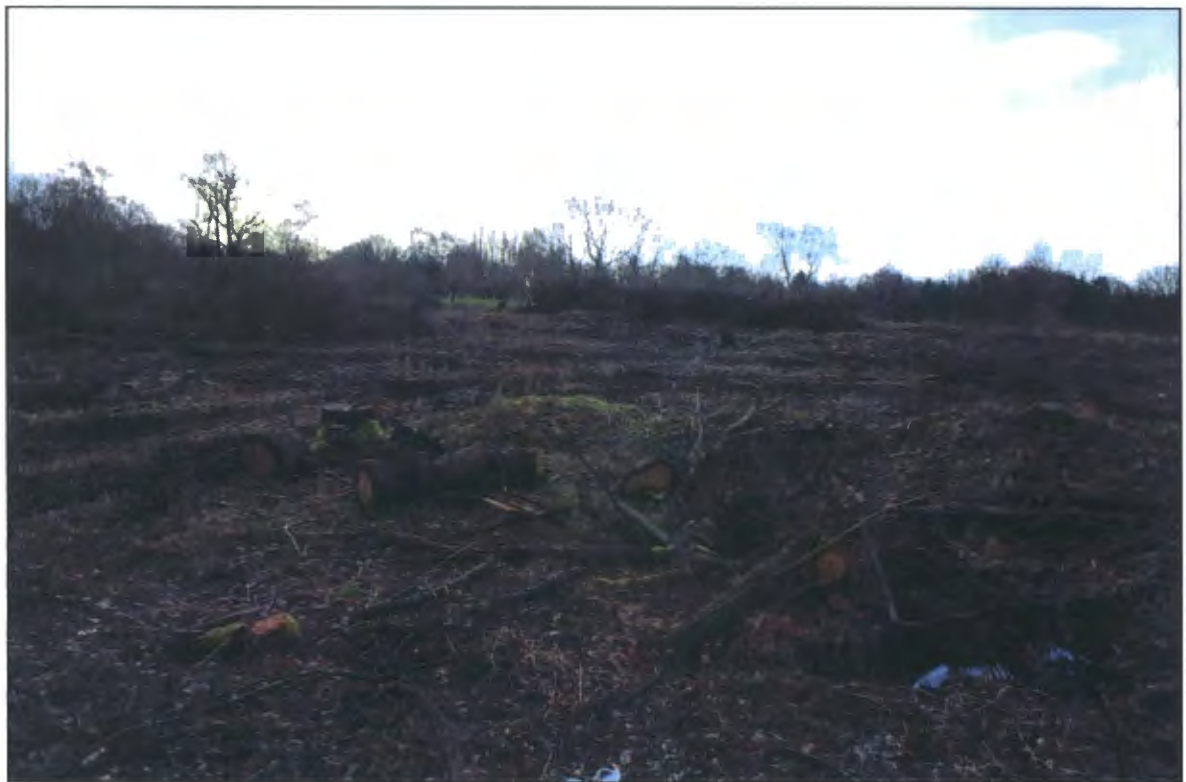
Plate 4. Piles of cleared timber.
