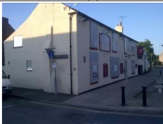
Photograph 1 Building from the south-west
