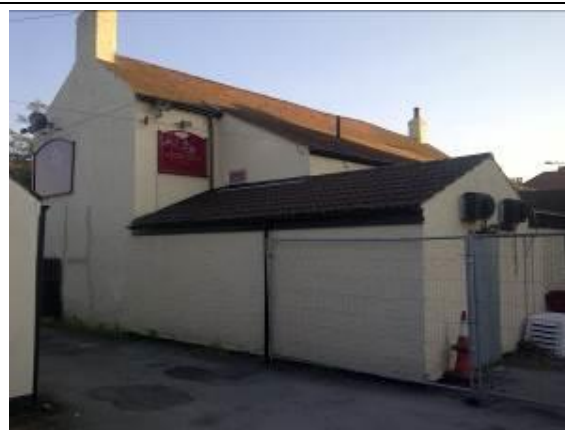
Photograph 2 Building from the north east
