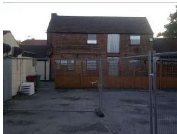
Photograph 3 Central storage building from the east.
