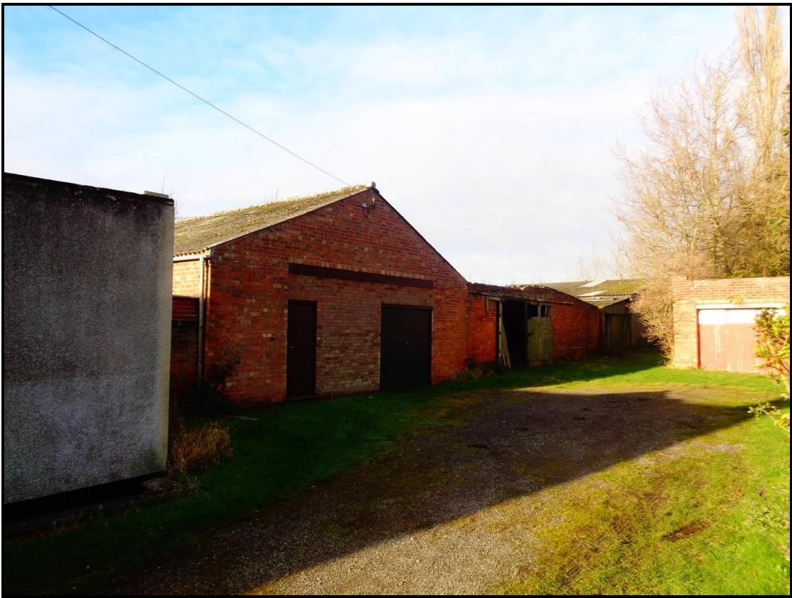
Existing Outbuildings to Rear
