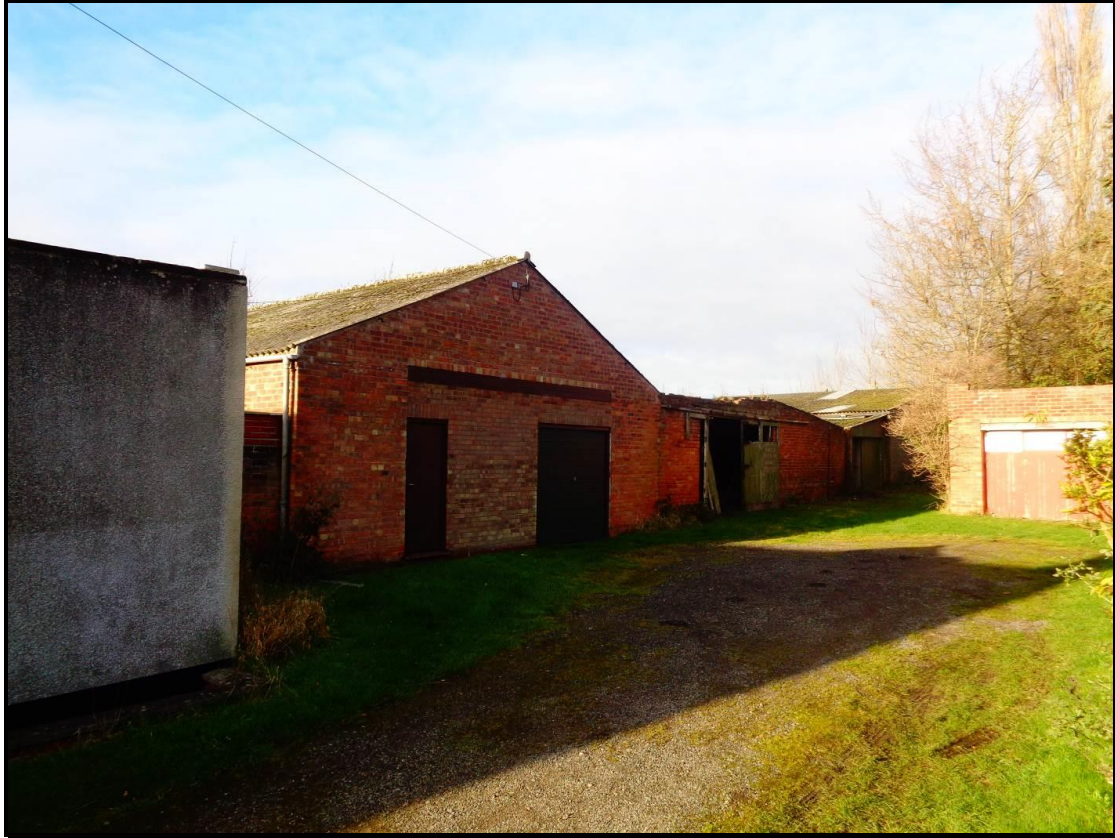
Existing Outbuildings to Rear of 7 Church Street, Showing East Elevation
