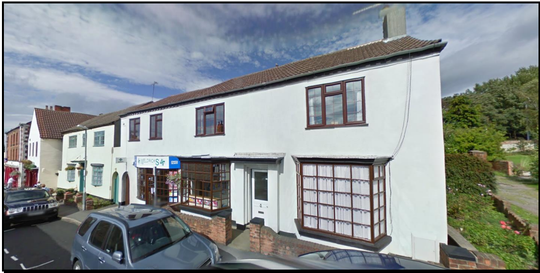
South Elevation of 7 Church Street
