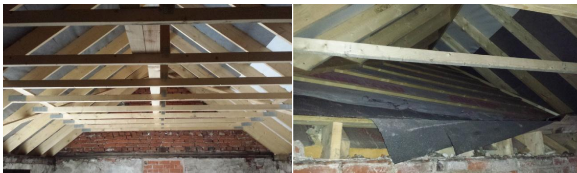
Photograph 4: Representative images showing the internal roof structure of Main Building.
