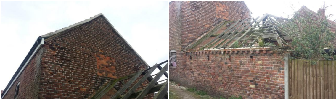
Photograph 2: Representative images showing the western gable end single storey extension.
