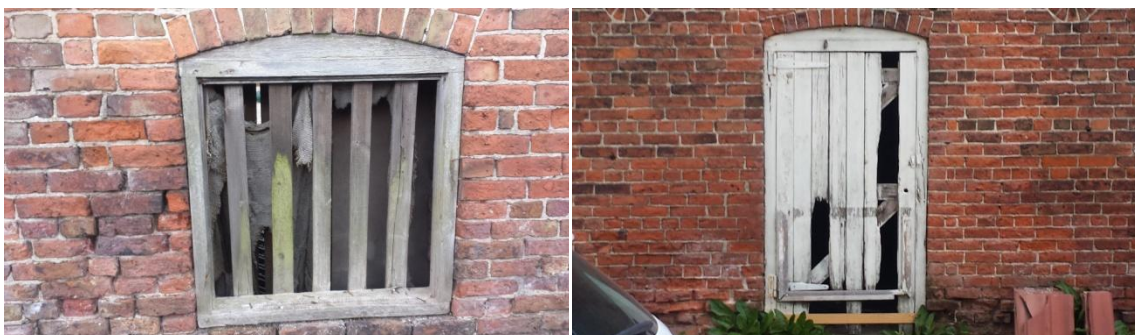
Photograph 3: Representative images showing a window (left) and ground floor door (right).
