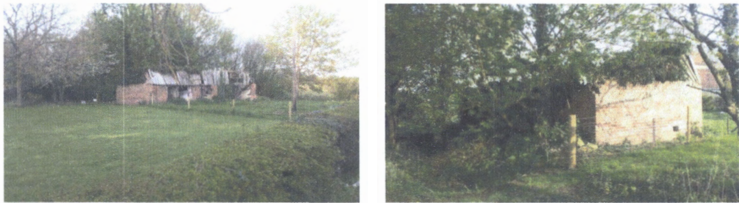
Photograph 5: Further representative images showing the external views of the outbuilding
