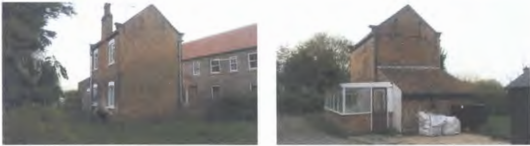
Photograph 3: Further representative images showing the exterior of Tetley Cottage
