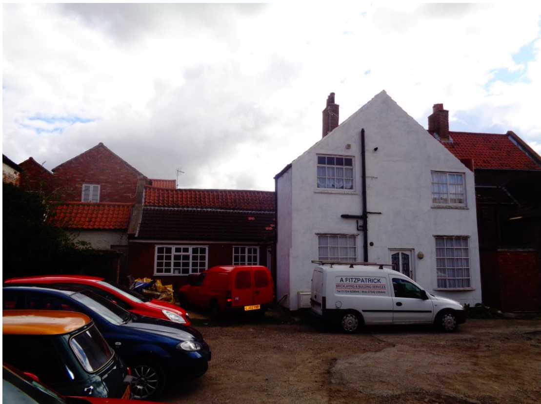
West Elevation (from adjacent car park)
