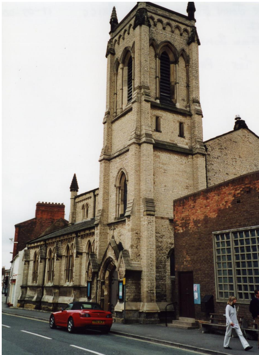
Adjacent Buildings of Townscape Merit
