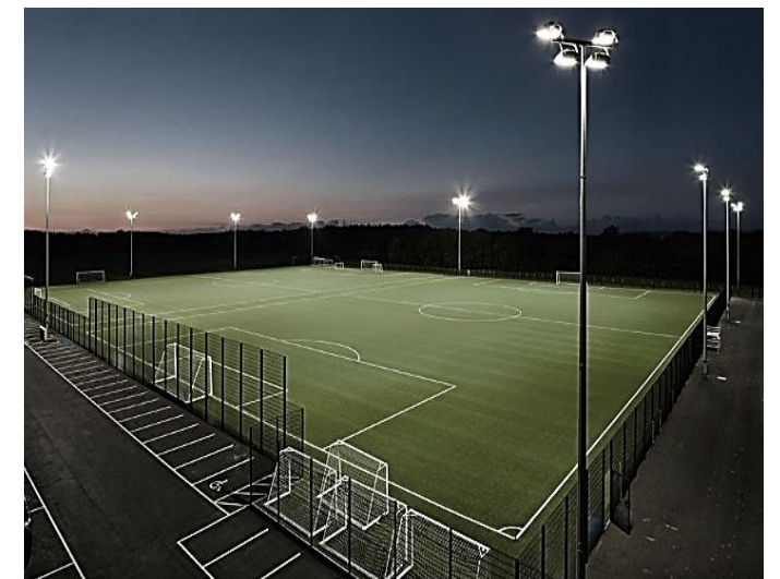
Typical 3G Artificial Grass Pitch (AGP) Installation
