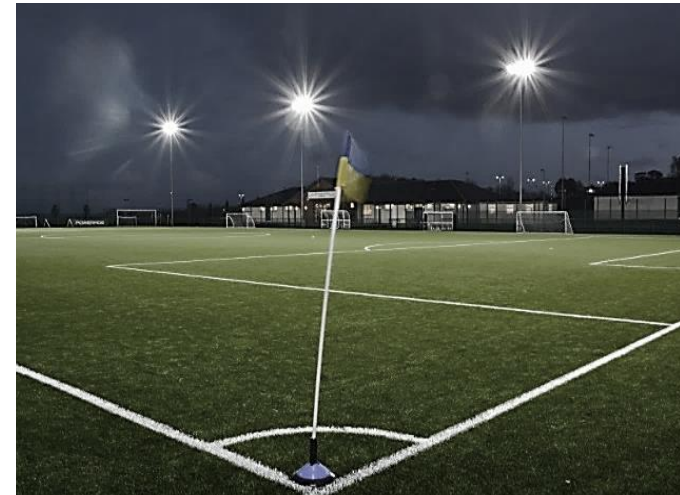
Typical 3G Artificial Grass Pitch (AGP) Installation
