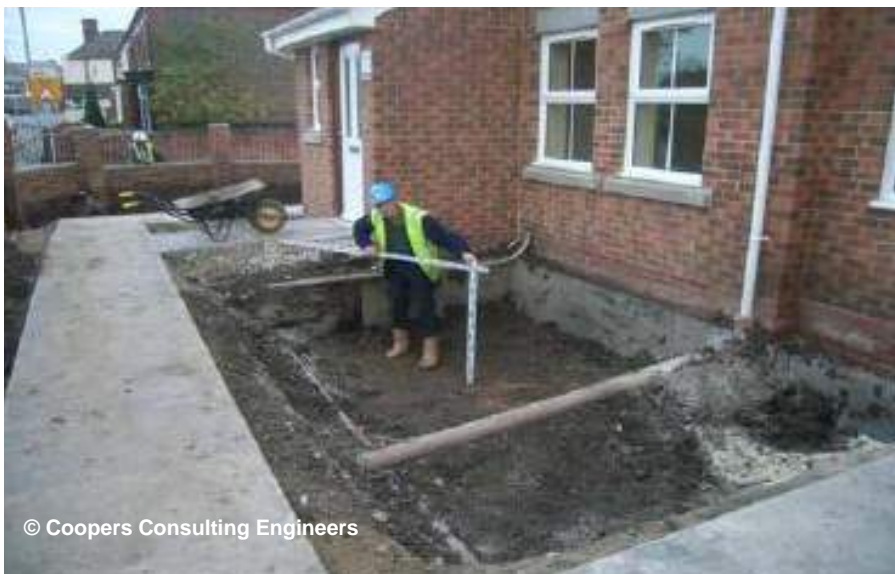
© Coopers Consulting Engineers
