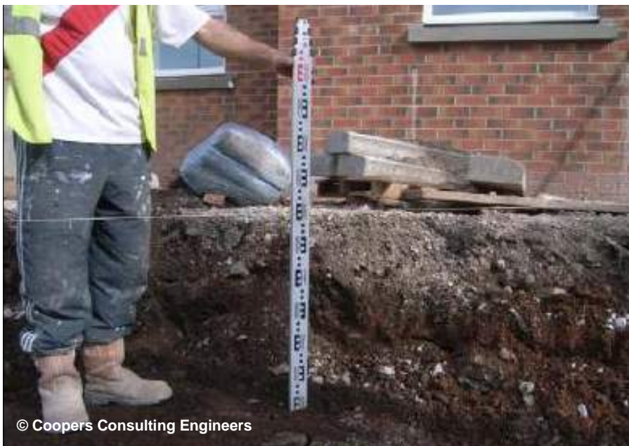
© Coopers Consulting Engineers
