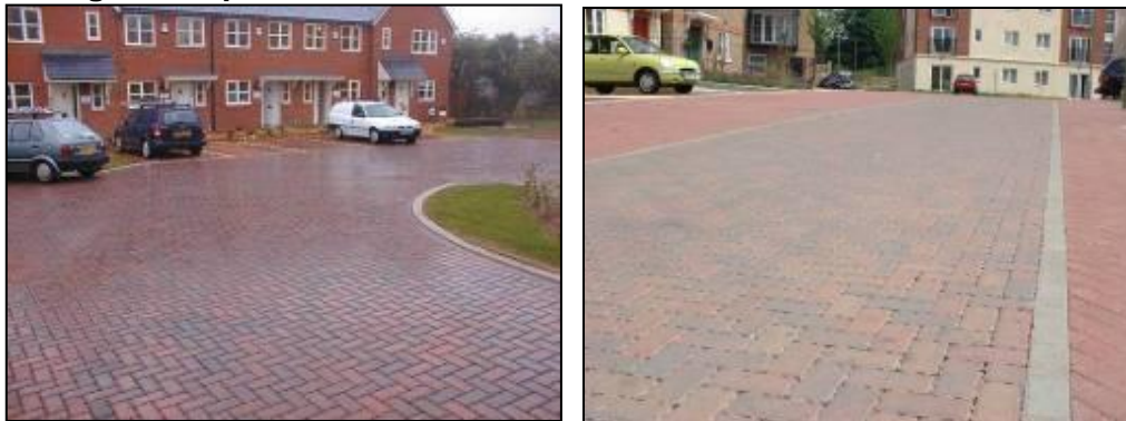
Meeting needs and requirements of PPG3 and PPG 25 Use of Priora on estate carriageways
