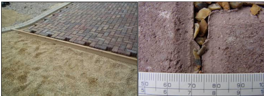
Priora Joint Fully Filled
