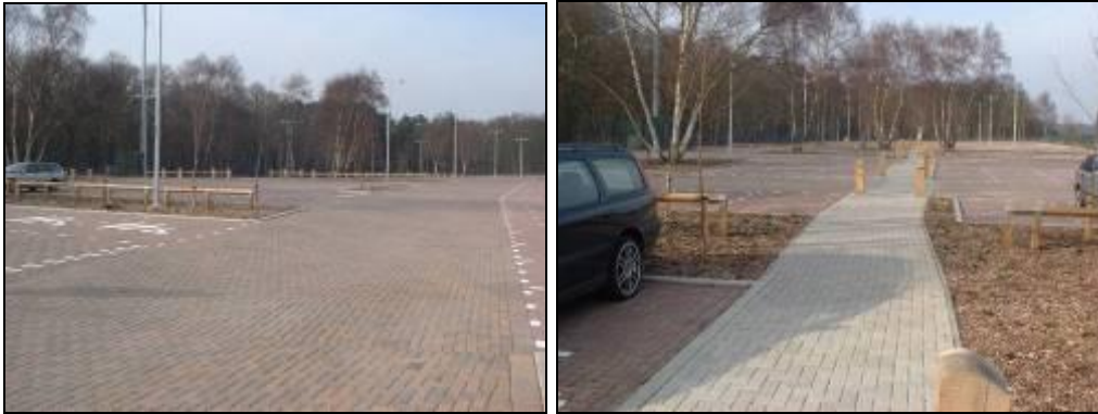
13,000 m2 continuously paved area.
