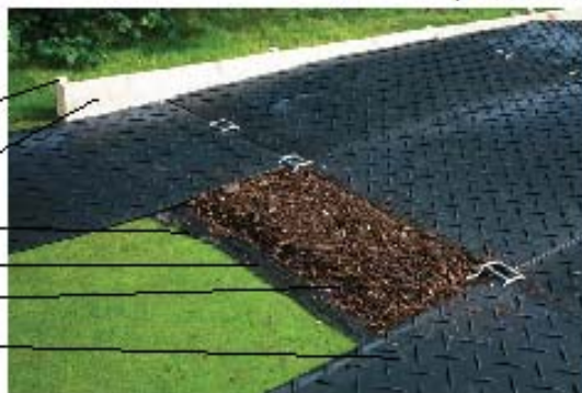
Ground-Guard trackways may be used with a cushion of woodchips to protect tree roots
