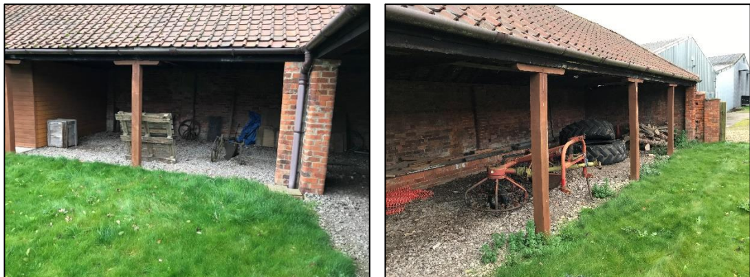
Photograph 1: Representative images showing the open-fronted elevations.
