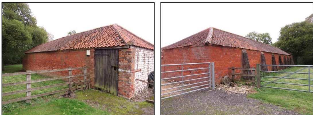
Photograph 2: Representative images showing the rear elevations.
