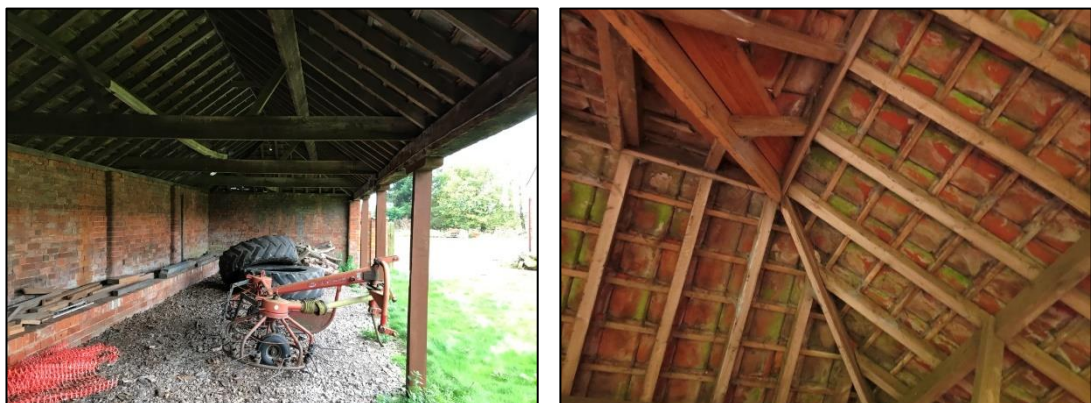
Photograph 3: Representative images showing the internal ceiling and roof apex.
