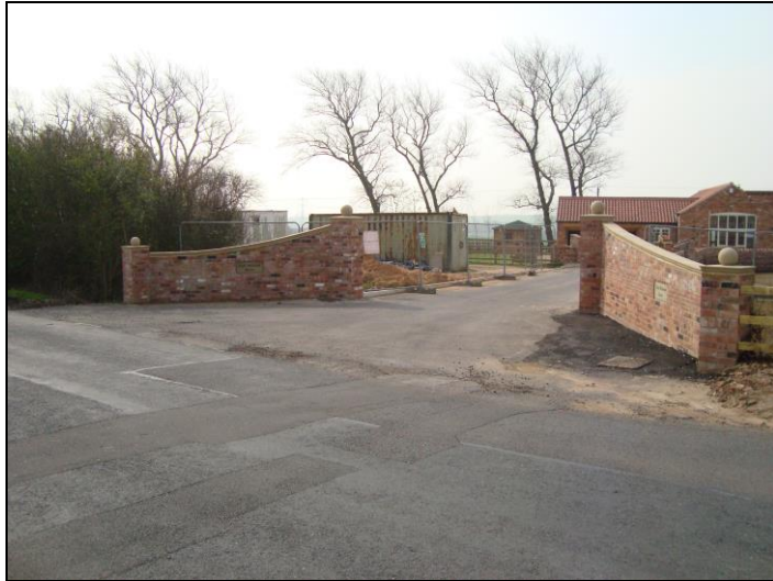
03. Existing Entrance to High Melwood Barns from Epworth Road.
