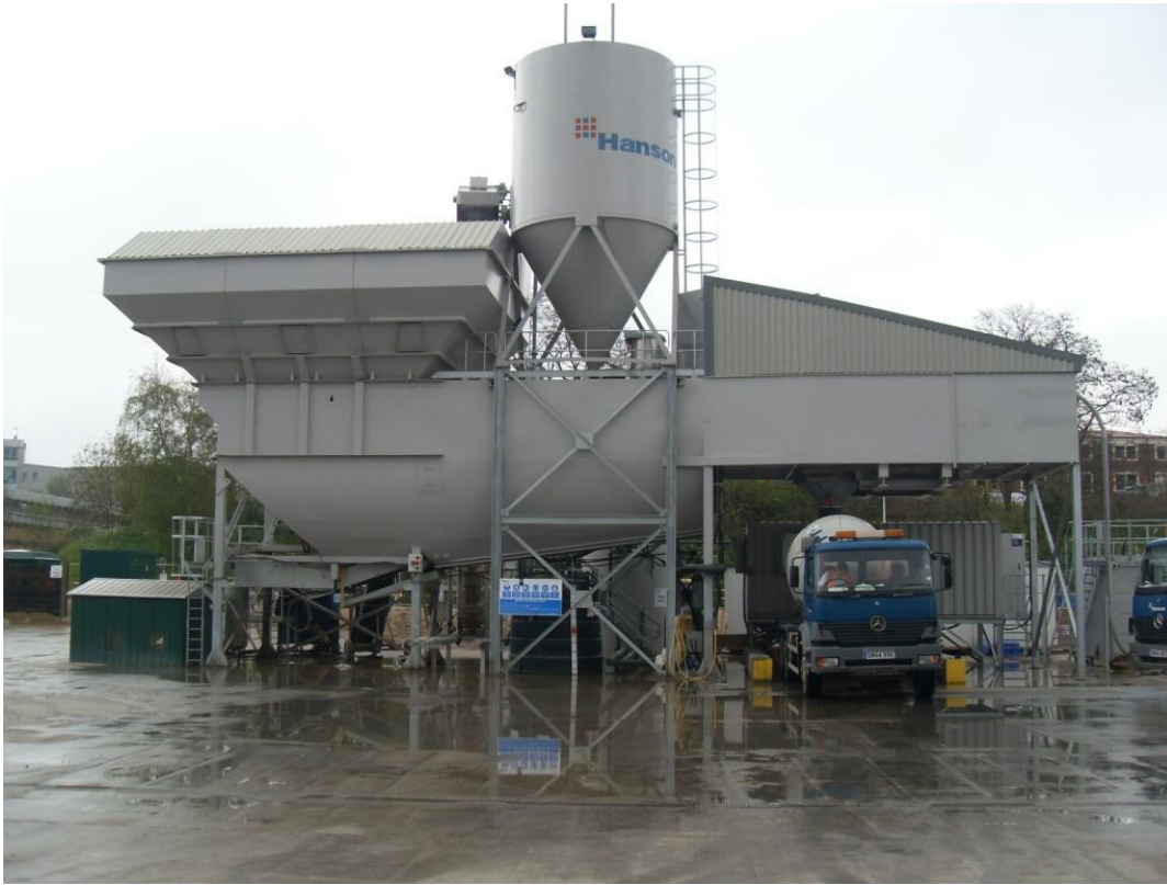
Steelfields Major 60 Old Oak Common Precast Facility
