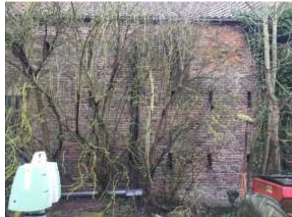
Figure 16: North elevation of barn obscured by vegetation with blocked pitching hatch
