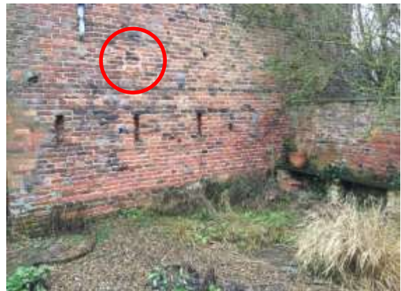
Figure 18: Brickwork to east elevation with blocked beam socket highlighted
