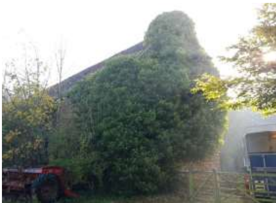
Figure 17: Ivy covering west elevation
