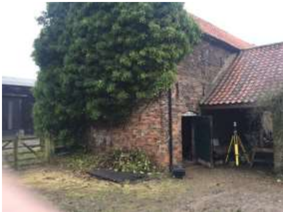
Figure 15: Abutment of horse mill with barn to south elevation
