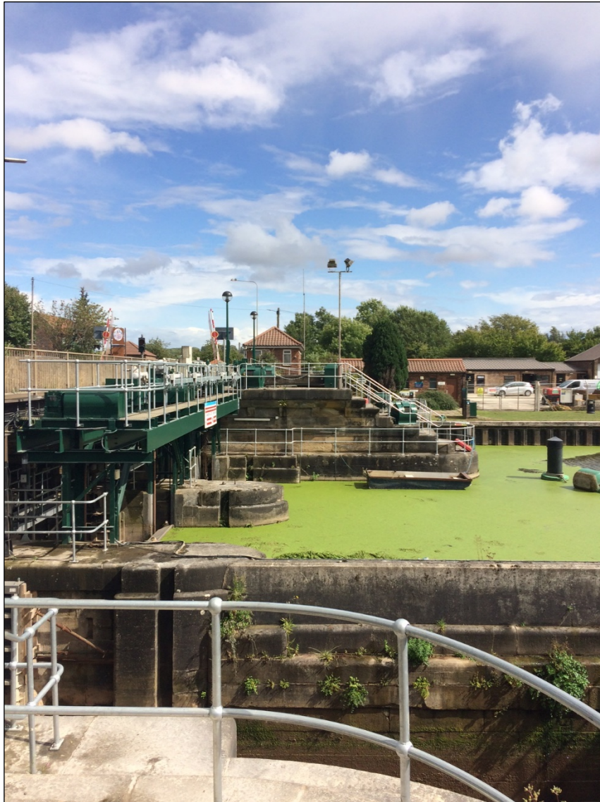
Plate 1: View of Ferriby Sluice (NHLE 1005244) from west
