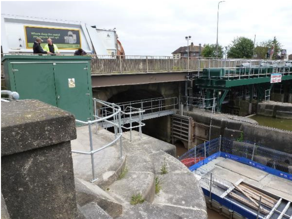
Photograph 13: Ferriby sluice, looking north-east
