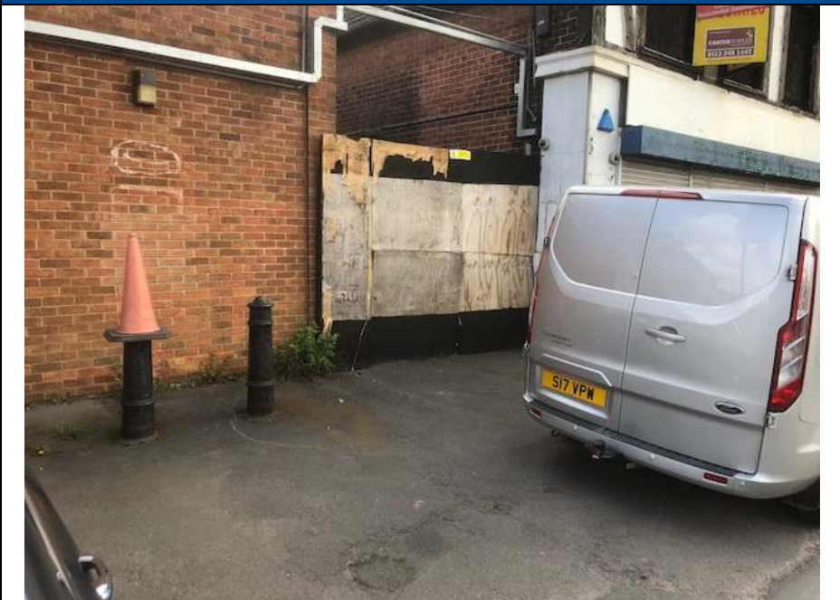
HYGIENE UNIT POSITIONED BEHIND HOARDING
