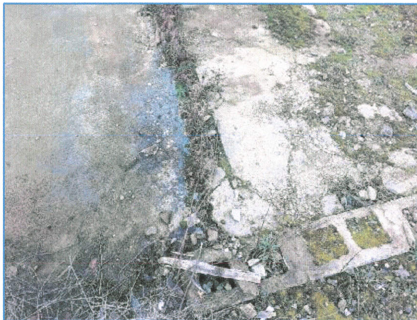
Slab to the LHS of entrance
