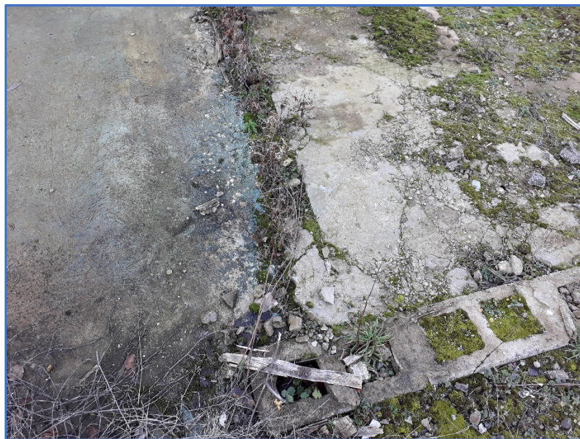
Slab to the LHS of entrance
