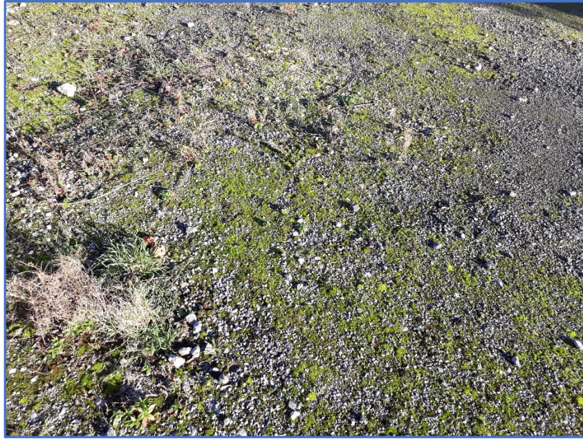
Hardstanding middle of site
