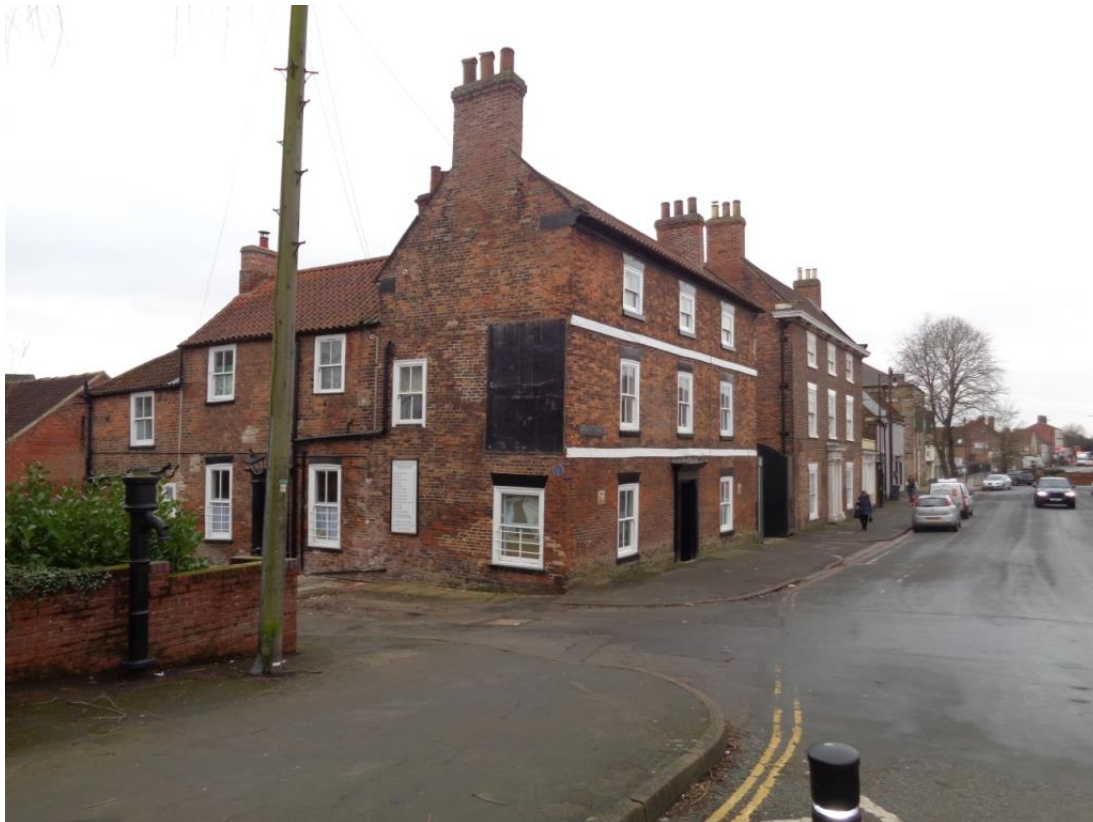
Looking South West at the North Eastern Corner of the Front Elevation of the Nelthorpe Arms
