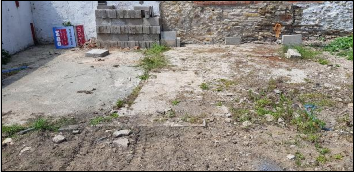
Southwest site corner and possible former bowser / tank storage area (view to west)
