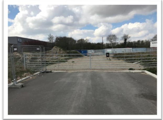
Photo 2: Extent of access road with gates to adjacent business. Proposed development is to the left of this picture.
