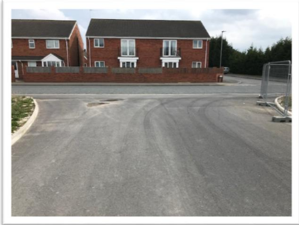
Photo 1: New junction and access road from Barton Road already constructed.
