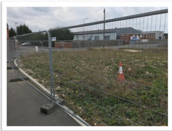
Photo 3: General state of site, with Heras fencing forming a temporary boundary. Access road and kerb visible to front of shot.
