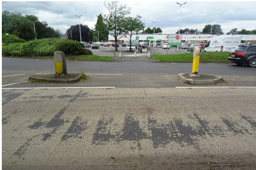
Photo 2: Pedestrian Refuge Island on Scotter Road
