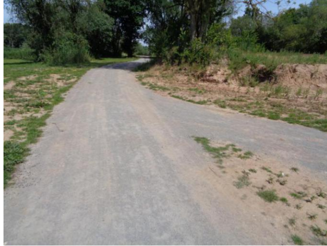
Hard surfaced track
