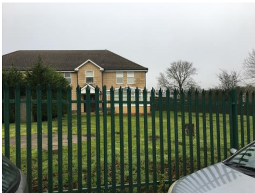
2.1 View of Rawton House from the car parking area
