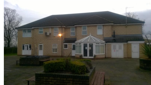
1.2 Existing North elevation of Rawton House, Options Roxby
