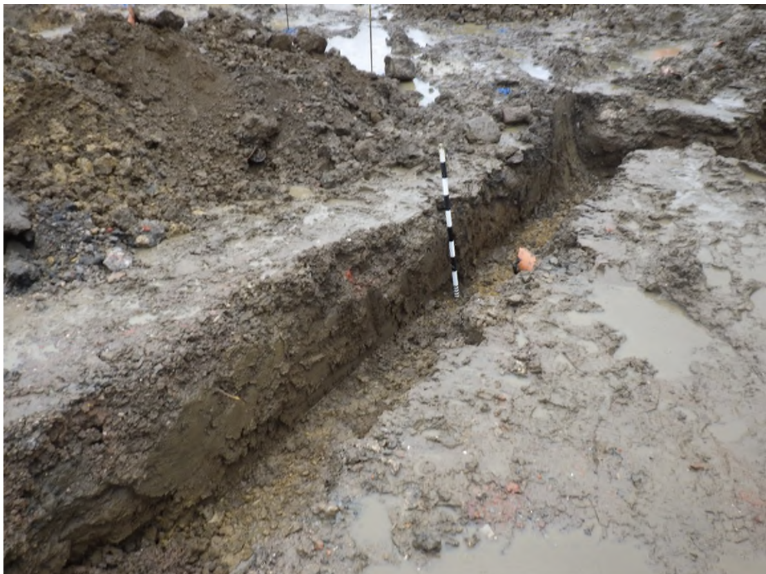
Plate 4 The southern side of the house foundation, showing deposit 5. Looking SW (1m scale).
