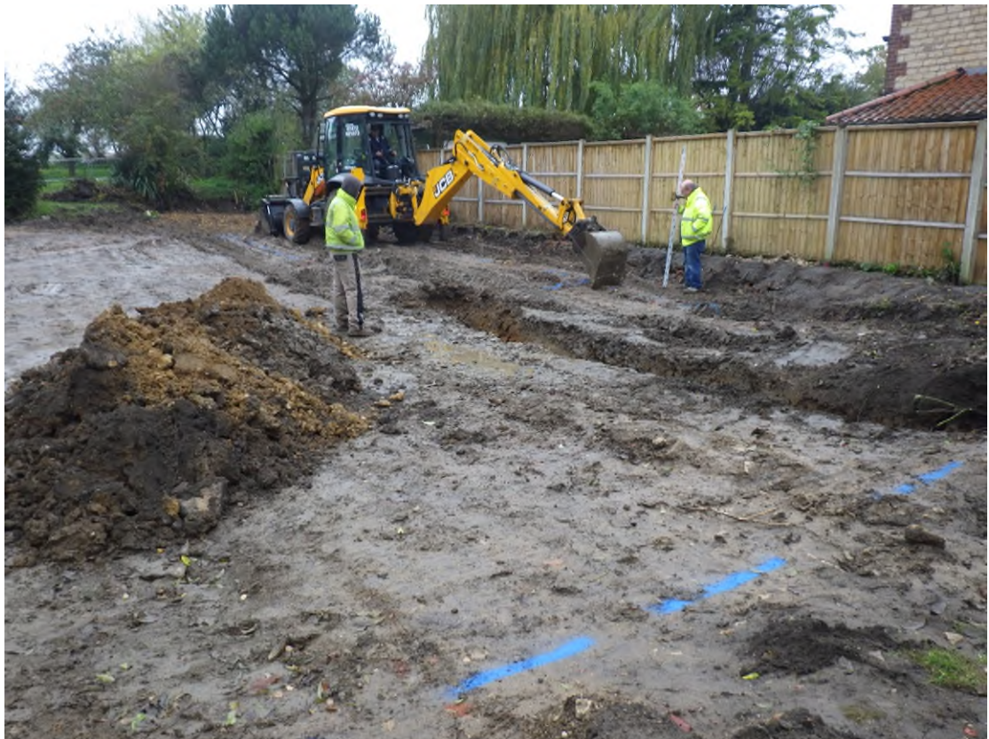
Plate 2 Initial excavation of the house foundation, looking west.
