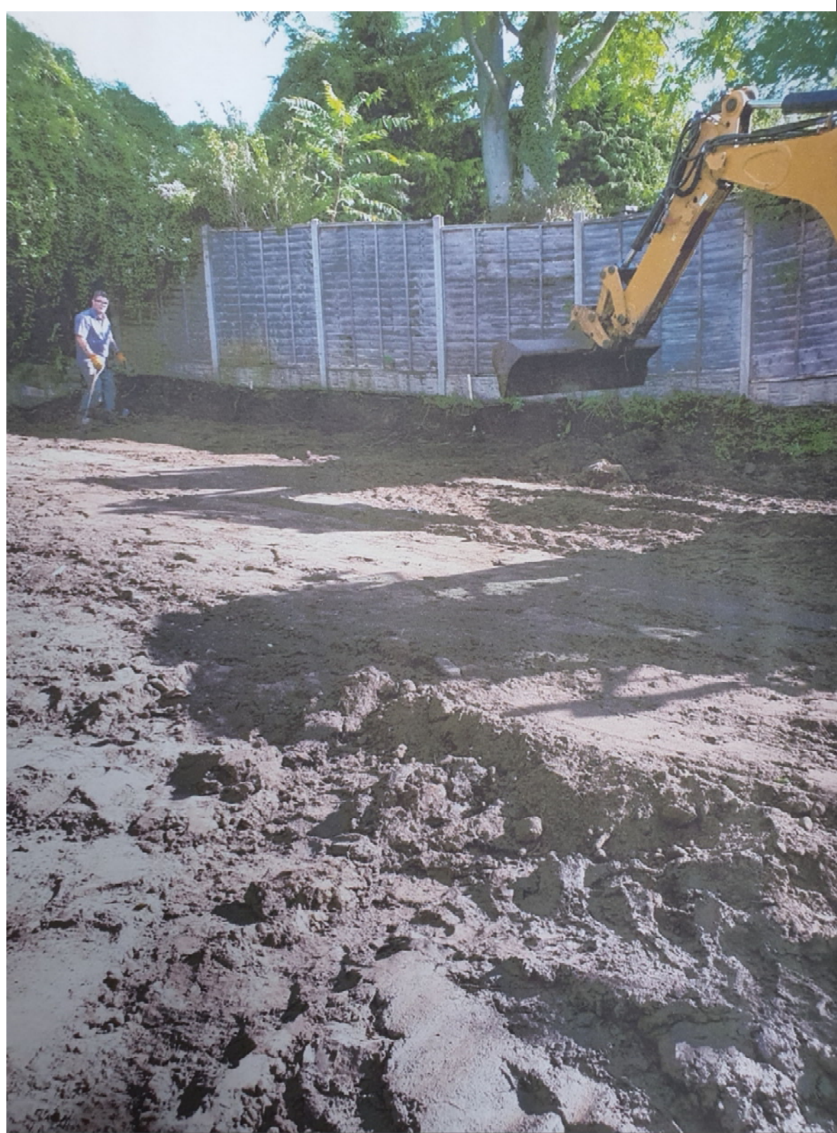
Made ground /soil removal from rear garden areas
