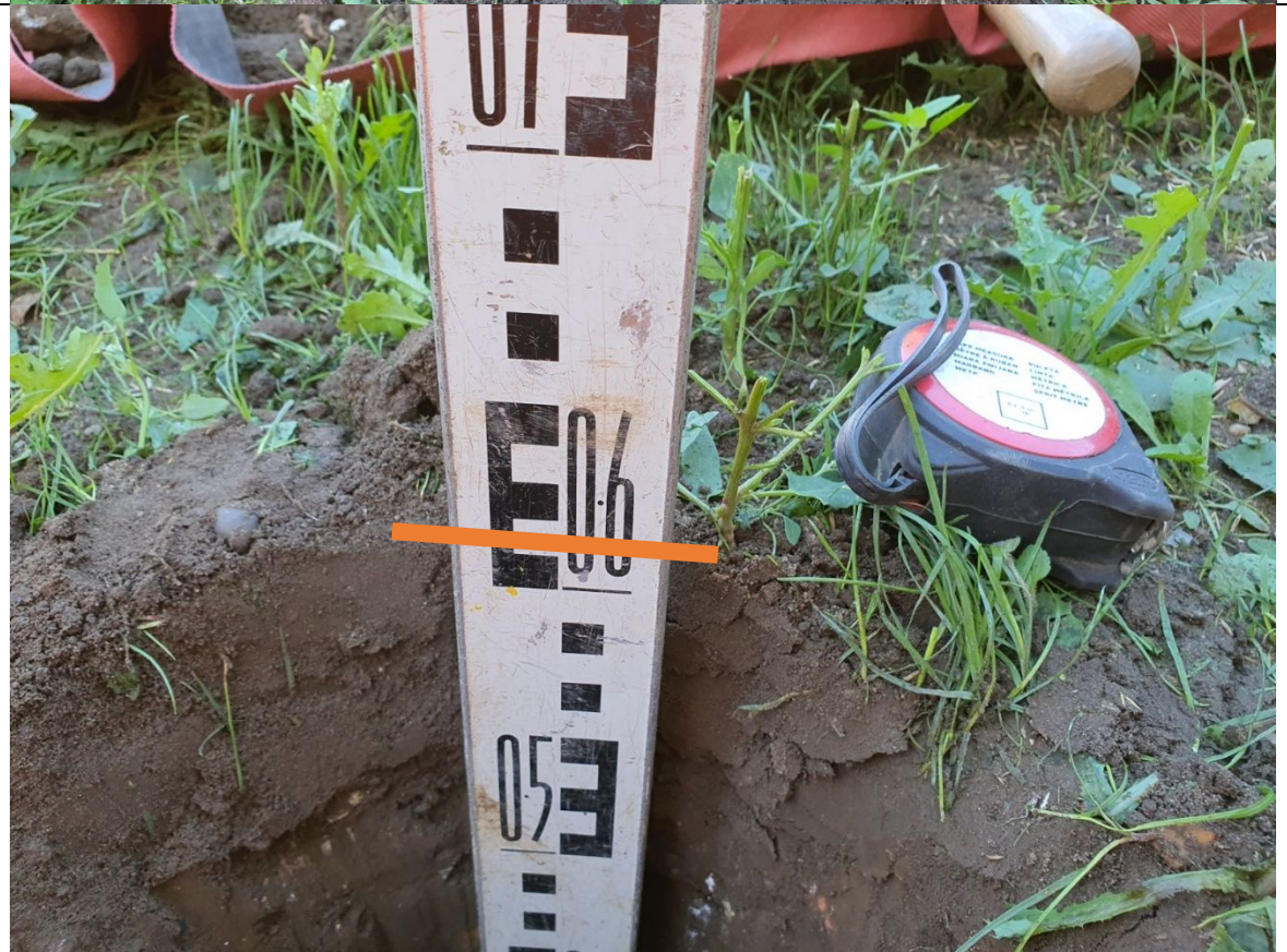
Trial pit 1 – rear garden granular capillary layer
