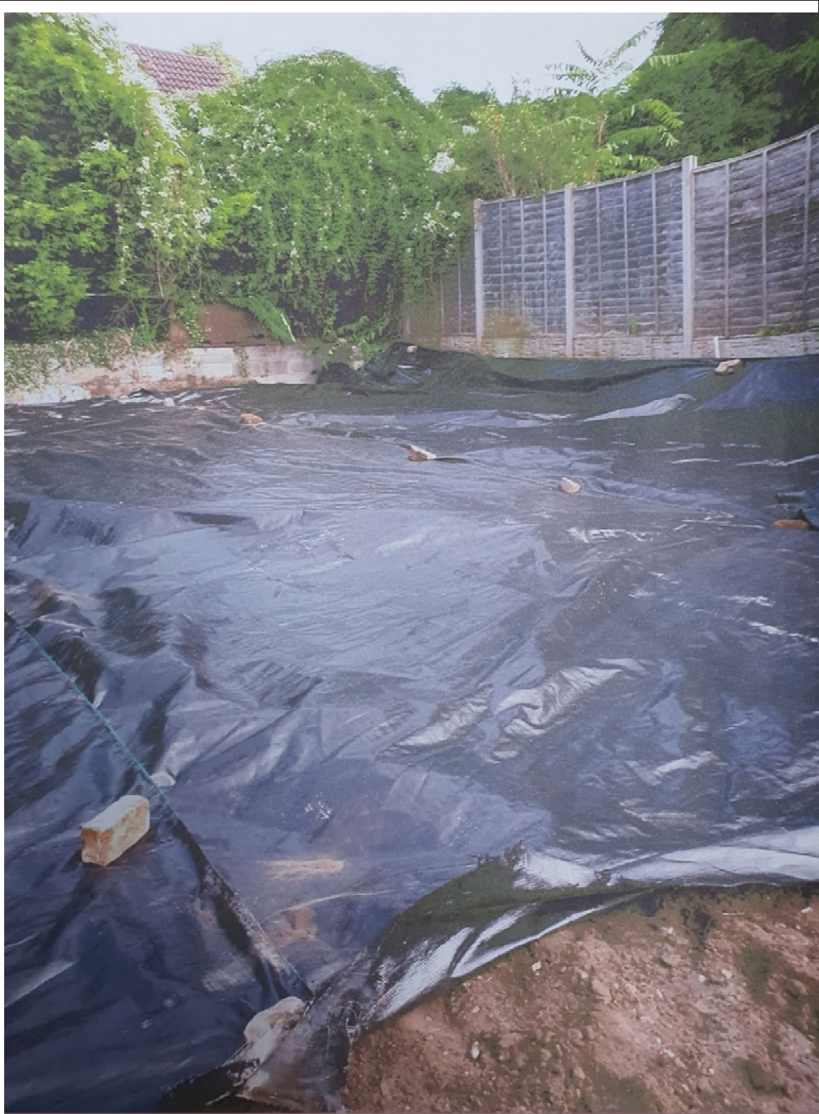
Placement of geotextile
