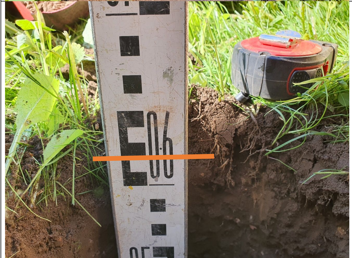
Trial pit 2 – rear garden granular capillary layer
