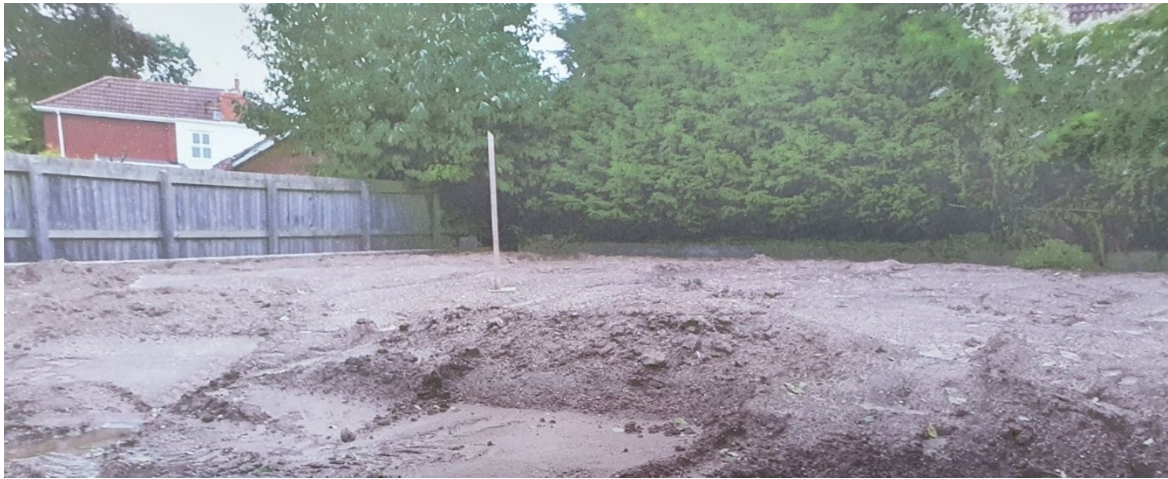
Placement of topsoil
