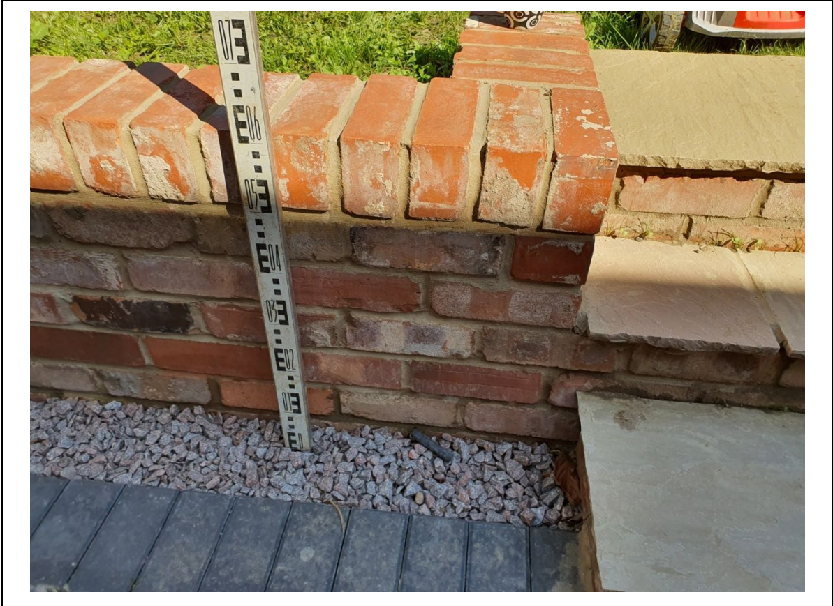
Construction of retaining wall
