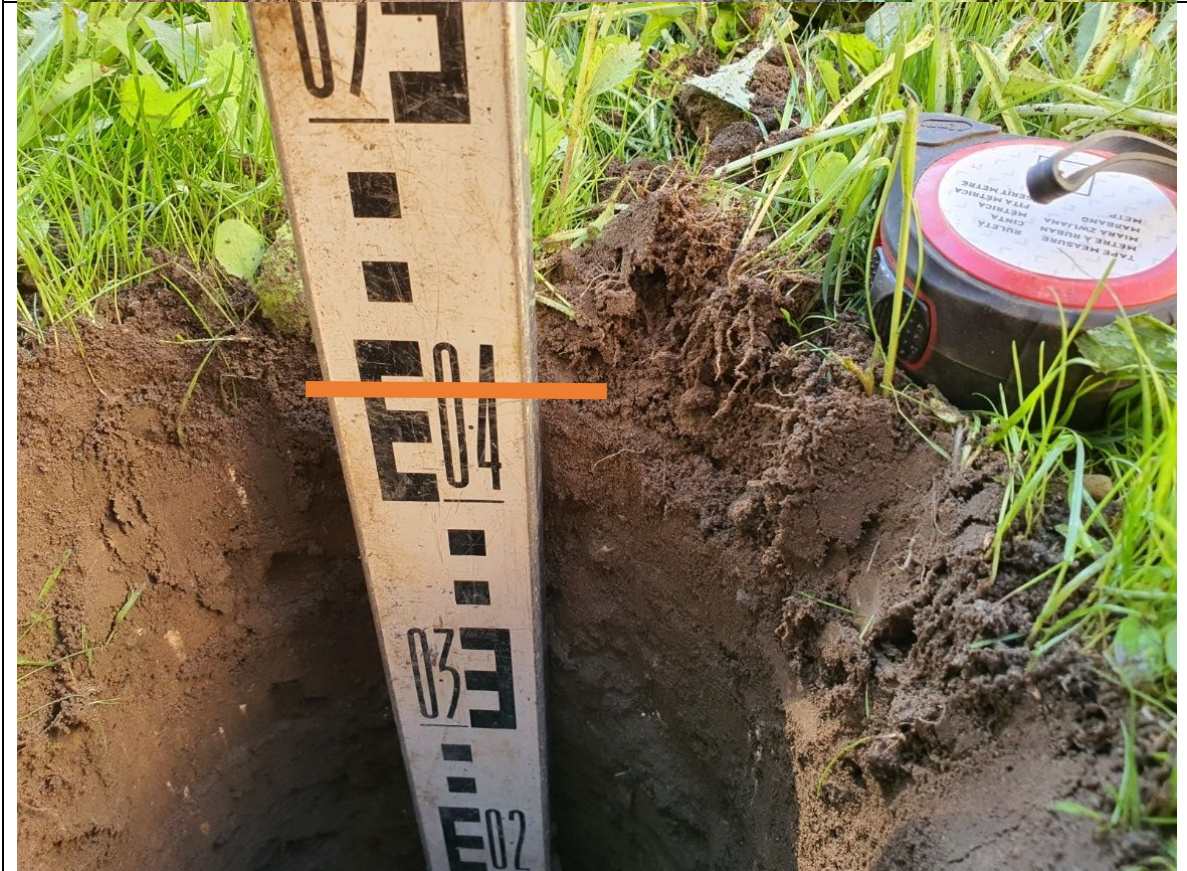
Trial pit 2 – rear garden topsoil
