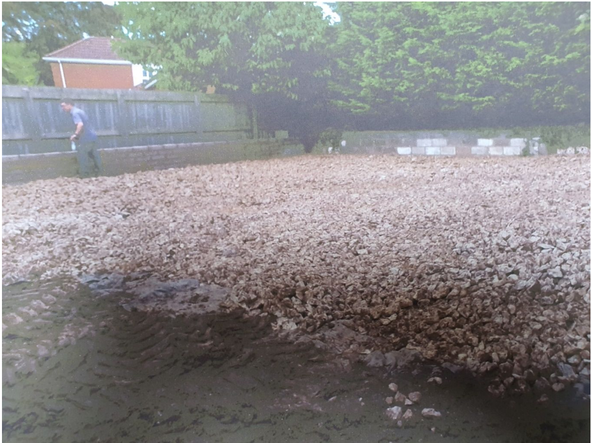
Placement of granular capillary break layer
