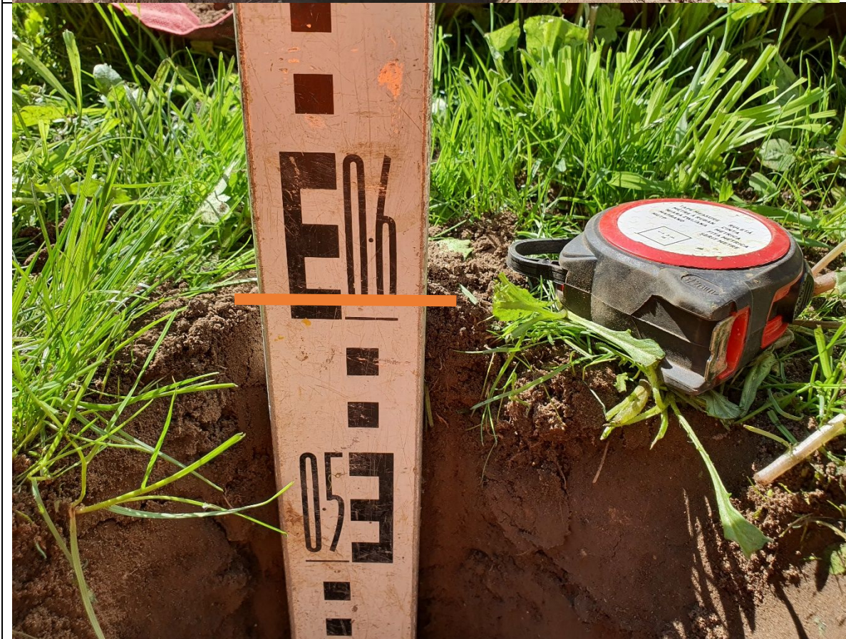
Trial pit 3 – rear garden granular capillary layer
