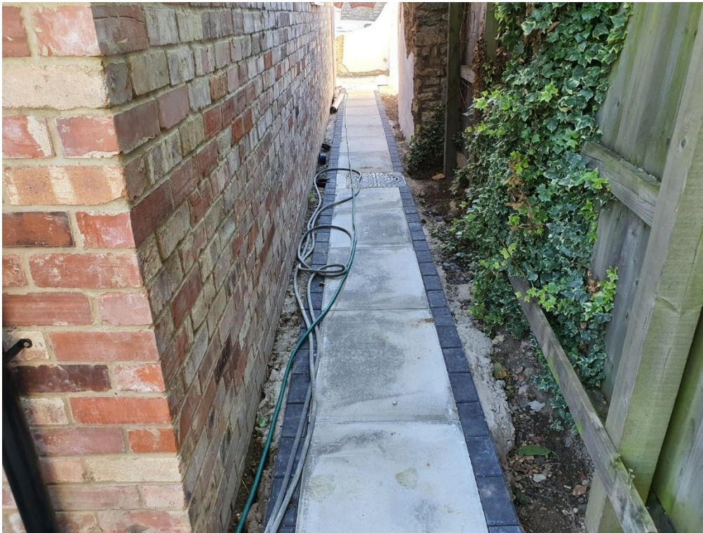
Plot 1 side walkway
