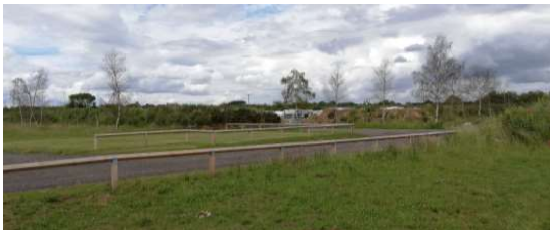
Photograph showing the secure gated access into the existing caravan and motorhome storage area consented in 2017, through which the proposed development site will be accessed.
