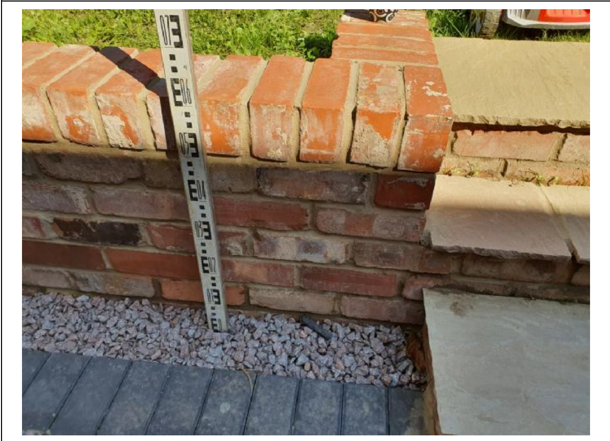
Construction of retaining wall
