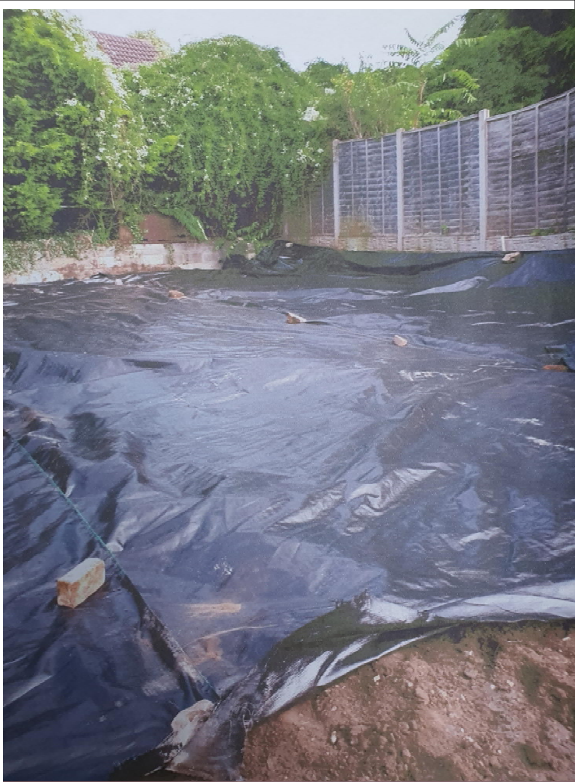
Placement of geotextile
