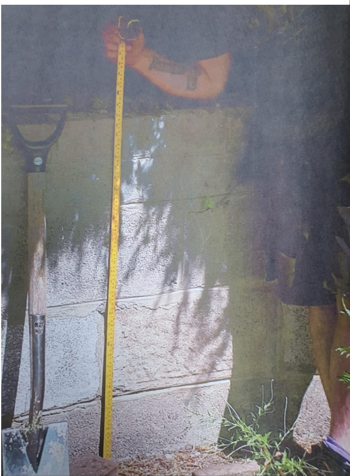
Evidence of level control
