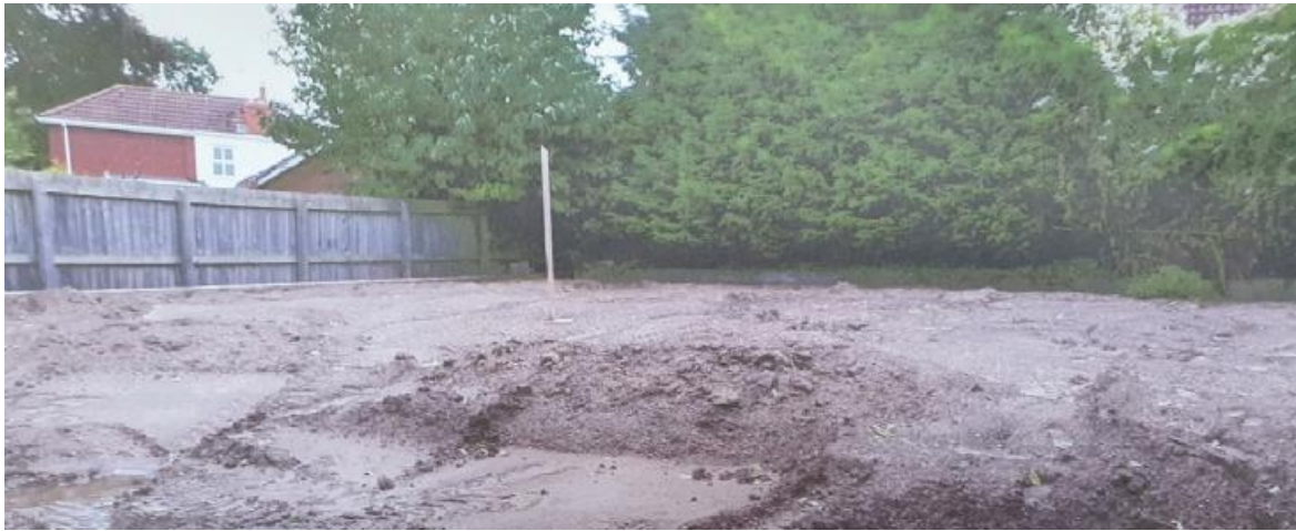
Placement of topsoil
