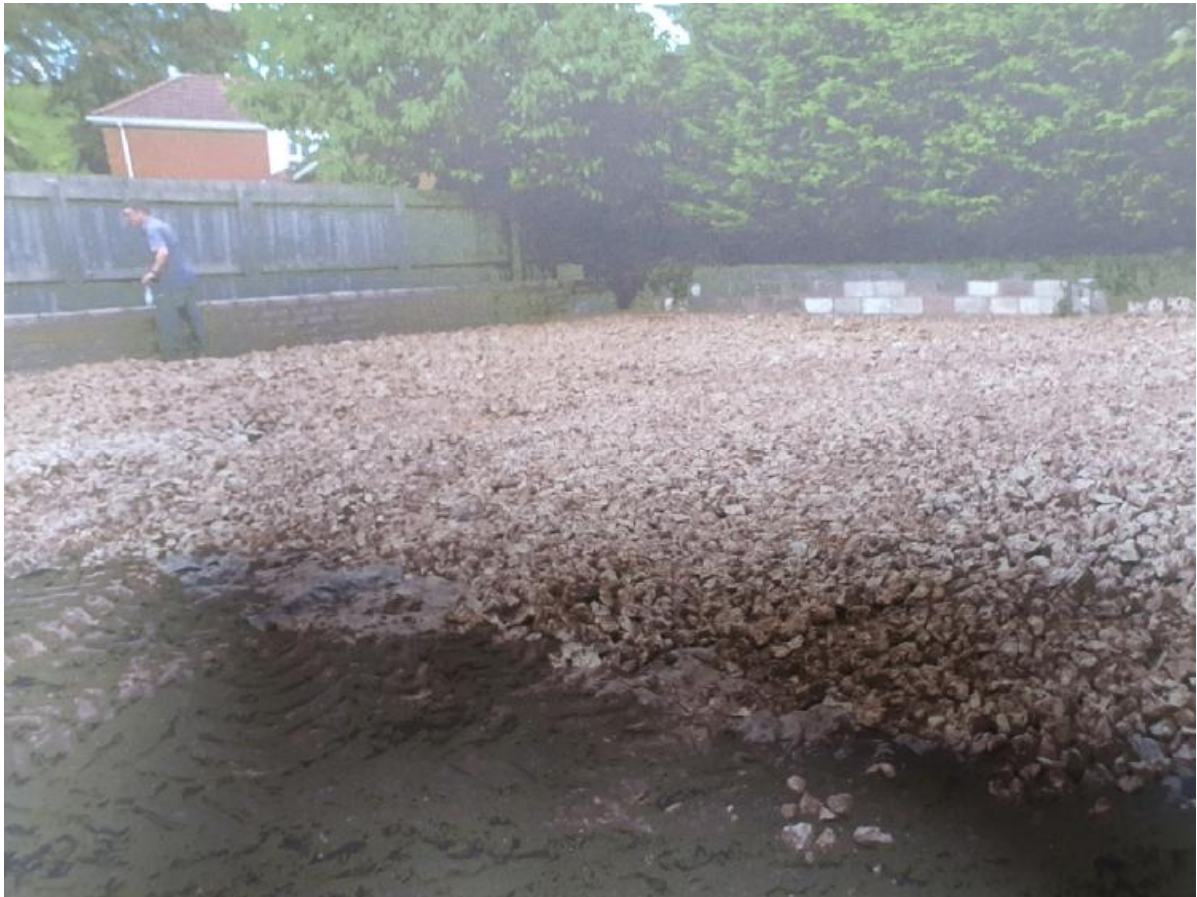
Placement of granular capillary break layer
