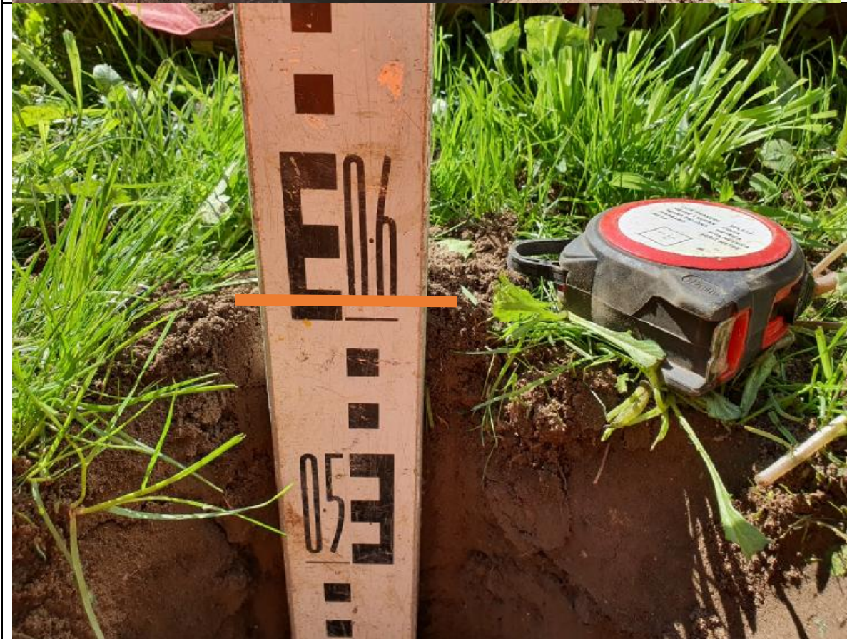
Trial pit 3 – rear garden granular capillary layer
