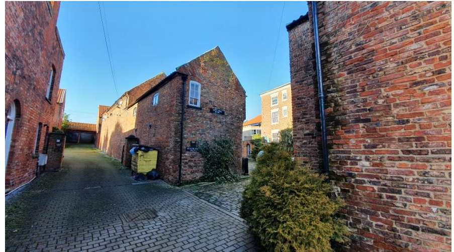
Figure Sixteen - View of adjacent properties with long gardens and outbuildings
