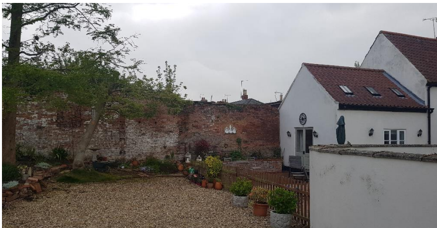
Figure Six – View of existing wall, which was formerly part of an outbuilding, from within the site facing North.
