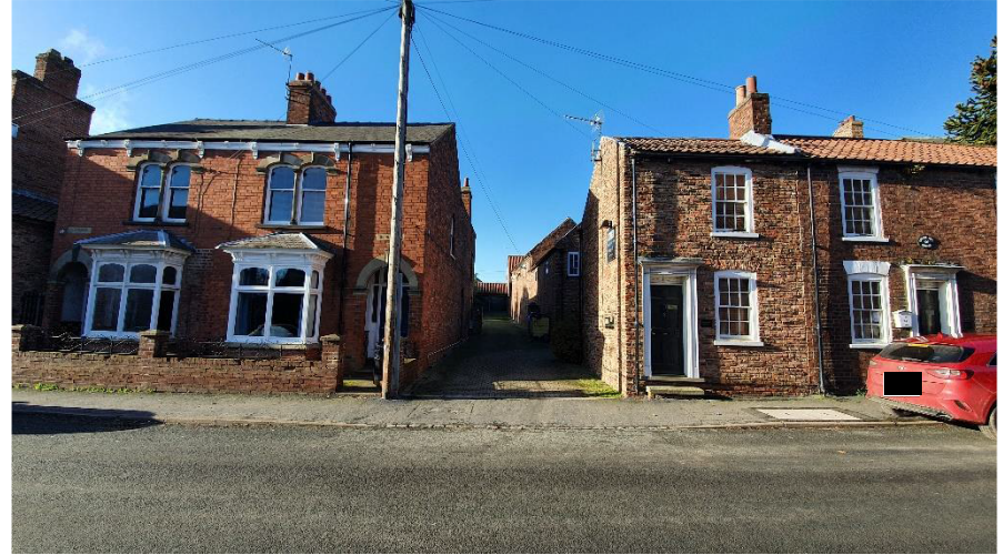
Figure Fifteen - View of adjacent properties with long gardens and outbuildings
