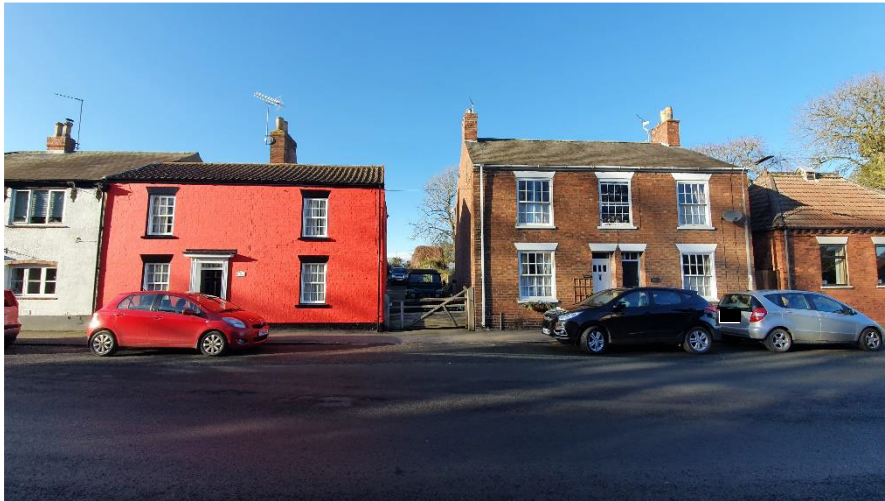
Figure Fourteen - View of adjacent properties with long gardens and outbuildings
